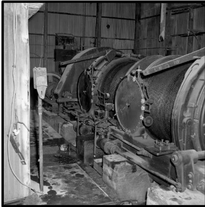
The abandoned Czar Mine hoist in 1963 (see p. 47, para. 3, p.57 para. 4 & p. 59 para. 6)
