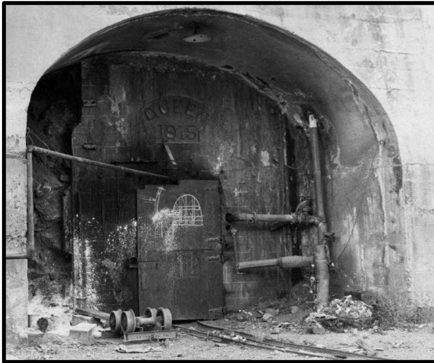
The Queen Tunnel/adit in 1963(see p. 24, para. 3 & p.30, para. 3)
