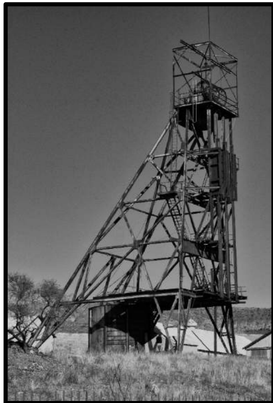
The remains of the Denn Mine headframe (see p. 101 para. 4)
