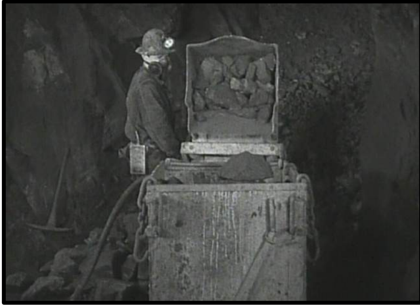
A miner loading a mine car with EIMCO mucking machine in the Campbell Mine (see p.73, para.7)
