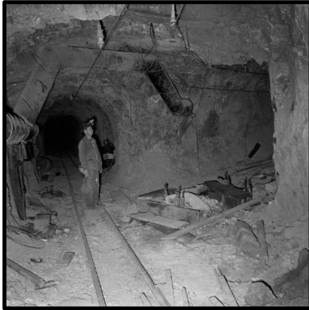
Lawrence Banks in the Cole Adit at a salvaged blower station in 1963 (see p.100, para. 2, p. 101 para. 5 & p. 104 para. 1)
