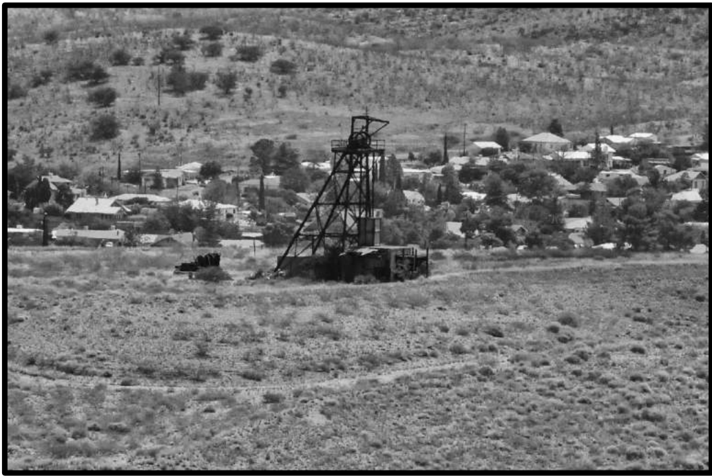
The abandoned Galena Shaft. This was an exploration shaft started by the Calumet & Arizona Mining company and was later taken over by Phelps Dodge. (see p. 69, para. 2 & p. 77, para. 4)
