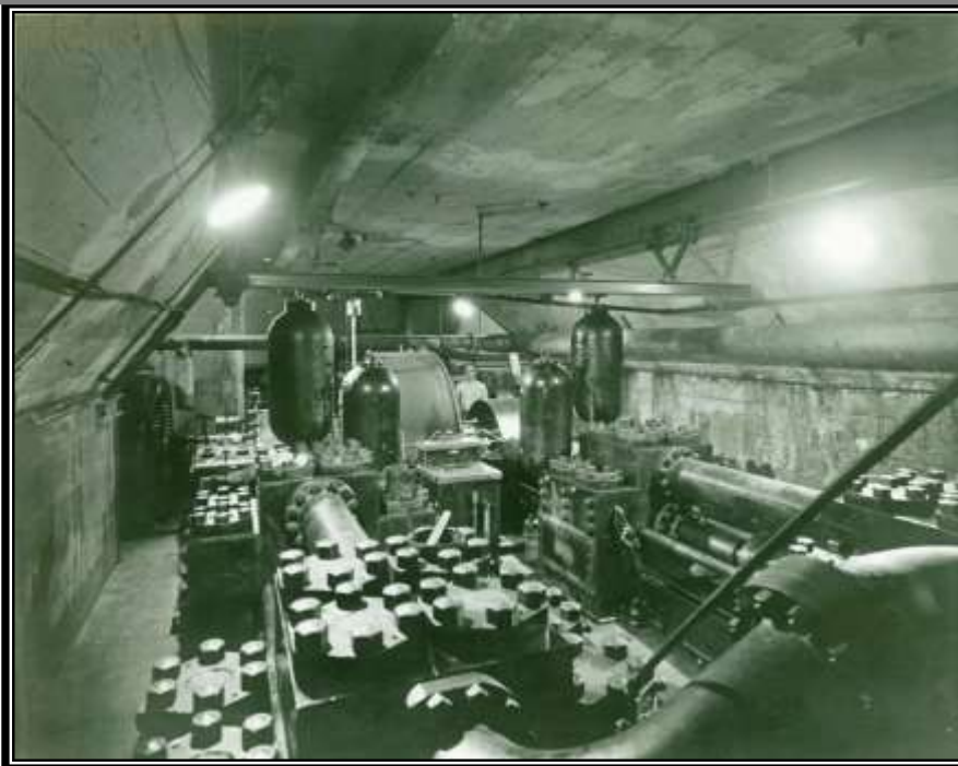
THE 2,250 GPM, # 6 PUMP, 2200 LEVEL JUNCTION MINE C - 1928
