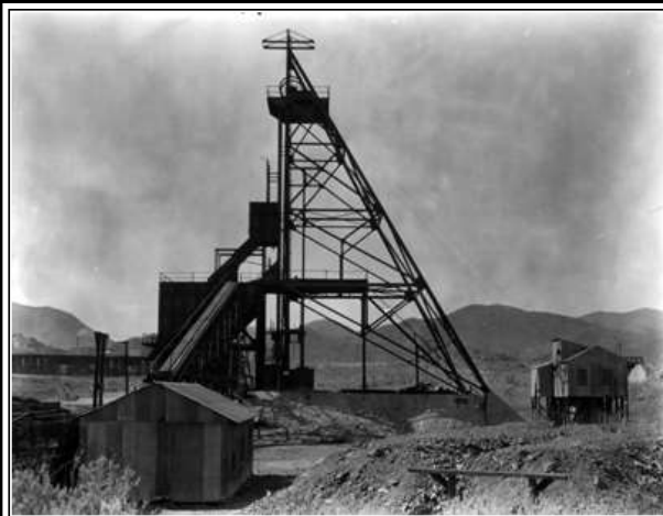
CAMPBELL MINE WITH THE INITIAL SINKING HOIST IN PLACE C - 1920
