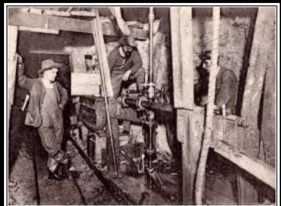
GRAEME LARKIN COLLECTION DIAMOND DRILL PROSPECTING IN THE C&A MINE - 1905
