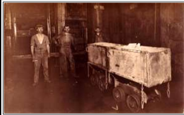
GRAEME LARKIN COLLECTION CAGE LOADING ORE CARS AT A SHAFT STATION C - 1908
