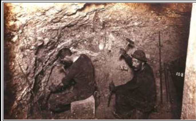
GRAEME LARKIN COLLECTION SINGLE JACK, HAND DRILLING IN A STOPE C - 1903
