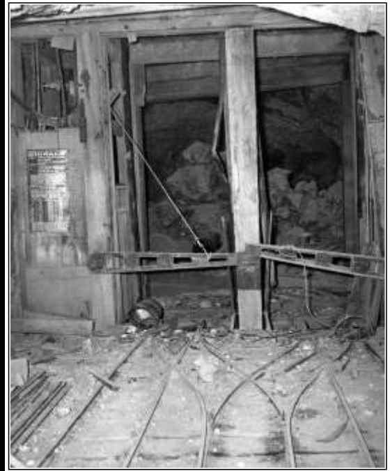
GRAEME LARKIN COLLECTION 400 LEVEL STATION, POWELL SHAFT - 1961
