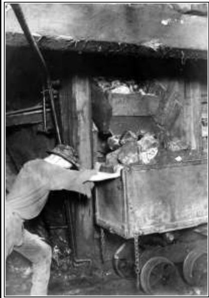
GRAEME LARKIN COLLECTION HAND TRAMMING LOADED MINE CAR C - 1915
