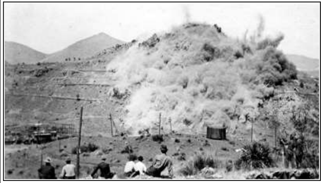
GRAEME LARKIN COLLECTION INITIAL BLAST ON SACRAMENTO HILL – JANUARY 1917
