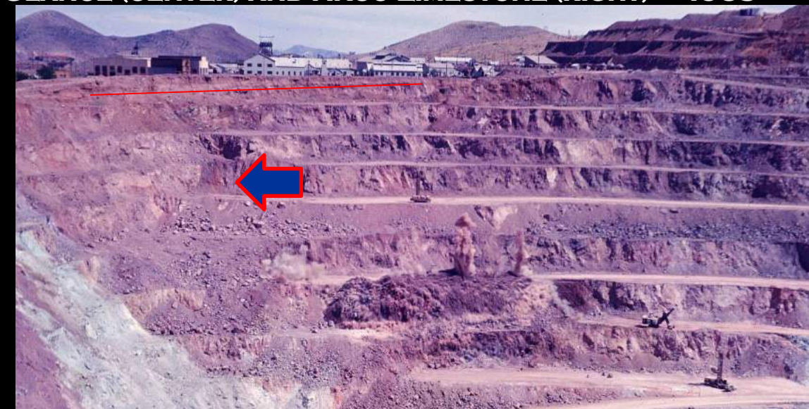
LOOKING SOUTHEAST WITH THE QUATERNARY SEDIMENTS ON THE GLANCE (LEFT) -1967 ; NOTE THE COLLAPSING GLANCE
