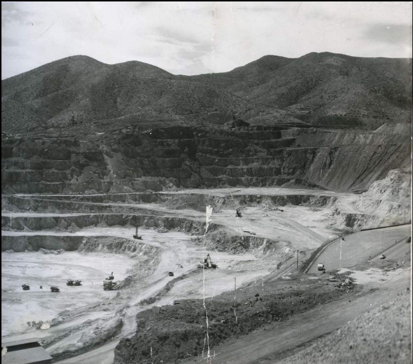
THE WEST END OF THE LAVENDER PIT, LOOKING SOUTHWEST IN 1957. THE HIGH WASTE DUMPS IN THE CENTER RIGHT ARE THE BACKFILLING OF THE SACRAMENTO PIT. SOME TURQUOISE BEARING MATERIAL WAS USED AS BACKFILL, GIVING THE INCORRECT IMPRESSION THAT TURQUOIS WAS FOUND IN THIS PIT AS WELL.
