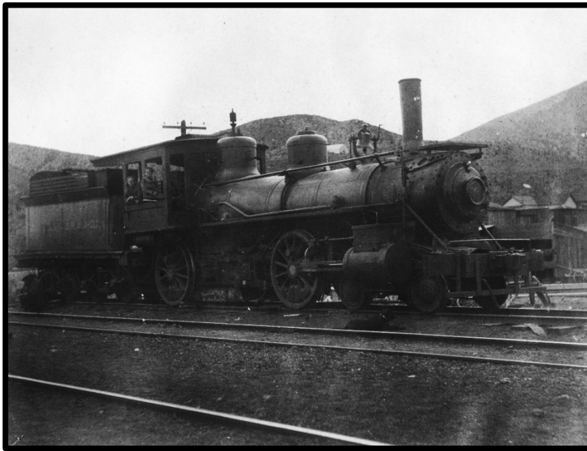
Arizona & Southeastern locomotive c-1900
