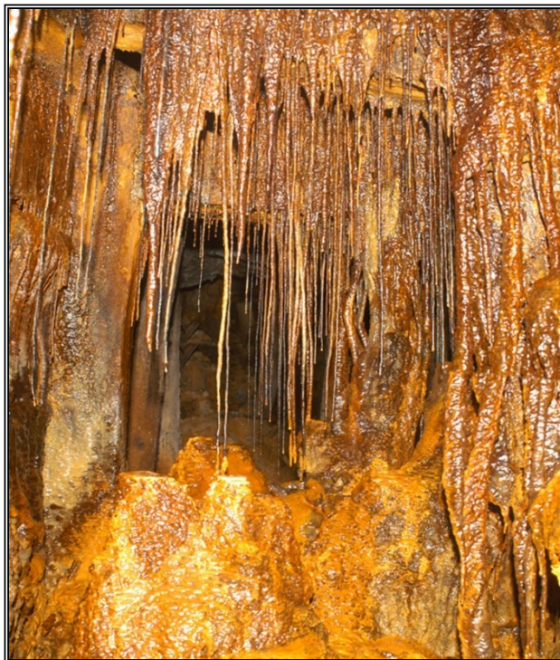
Iron hydroxide stalactites and stalagmites deposited by the acidic water that have partially filled the mine opening. 7 th level, Southwest Mine, vertical view—2.3 meters. Graeme/Larkin collection.
