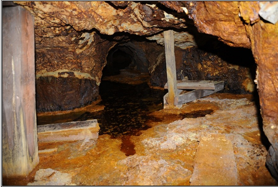
Ponded acidic mine water depositing iron hydroxide muds in abandoned working, note abundant white to brown melanterite on ceiling and walls, 6 th level, Southwest Mine, horizontal view – 2.8 meters. Graeme/Larkin collection.
