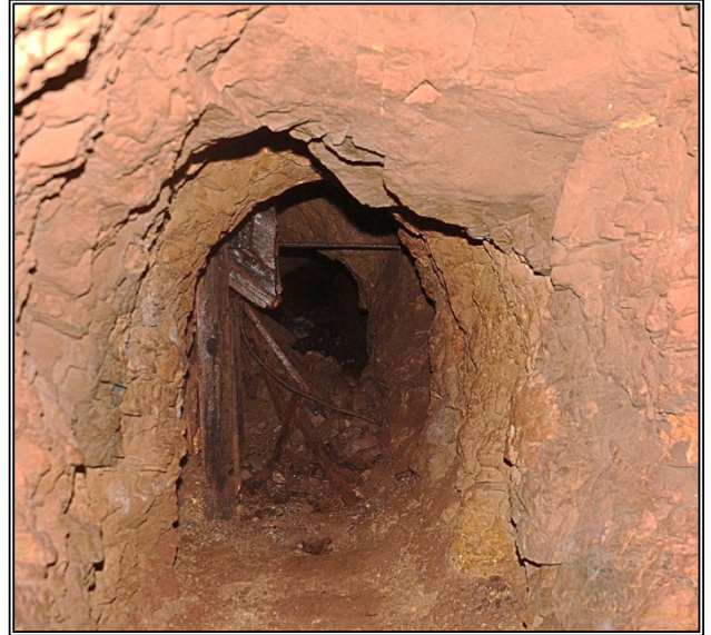
A typical, limestone crosscut in rock not impacted by cave development. The chute near the end suggest that ore was mined above, as some goethite was present in this small area. This location is on the same level and about 60 meters from the location illustrated to the left. Horizontal view-2.2 meters.
