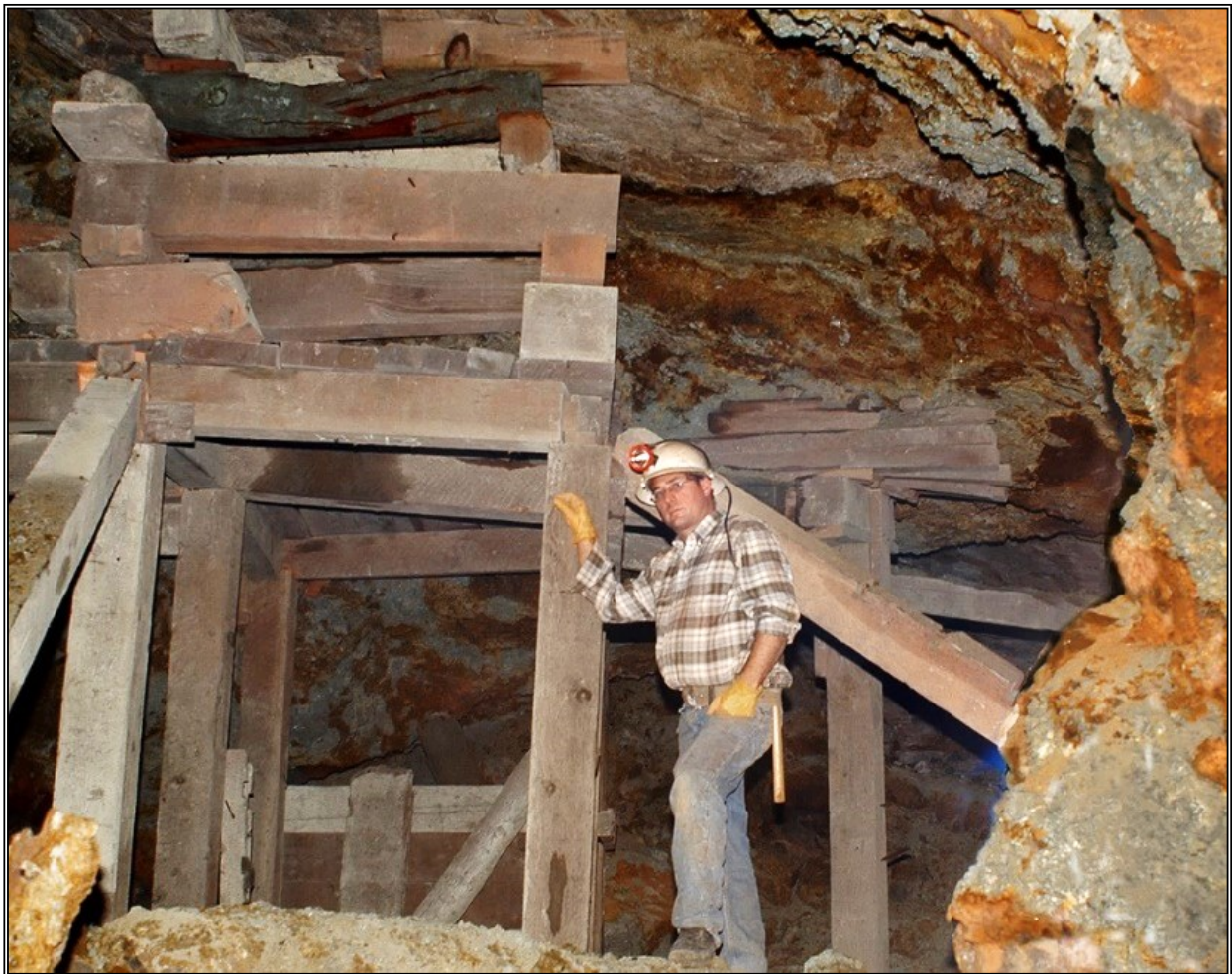
Oxidizing, low-grade pyrite shell that encased a sulfide orebody. Note the mine timber condition - almost like new - yet it had been installed more than 70 years before. The very dry, typically warm environment that is found with oxidizing pyrite has preserved the wood. One of the authors, RWG IV. is in the photo. 7 th level, Southwest Mine. Graeme/Larkin collection.
