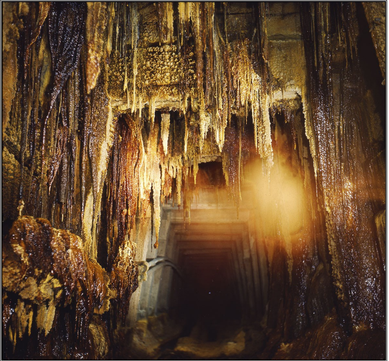
Post-mining iron hydroxides and melanterite coating mine timber. Some goethite is also present from the dehydration of various iron hydroxides. The location is on the 2833 level of the Campbell mine. 1973 photo from the Graeme/Larkin collection.
