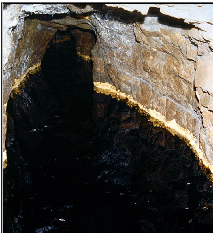
Left: Pondered acidic waters to 25 cm. deep, in a limestone crosscut, 6 th level, Southwest Mine, vertical view - 2.30 meters.
