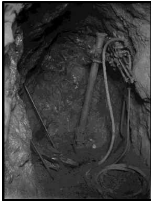
A safety photo showing an where a miner has drilled into a missed hole. C-1920
