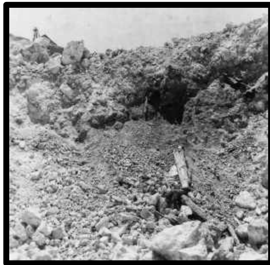
Timber from old underground mine workings in the wall of the Lavender Pit below the Gardner Mine
