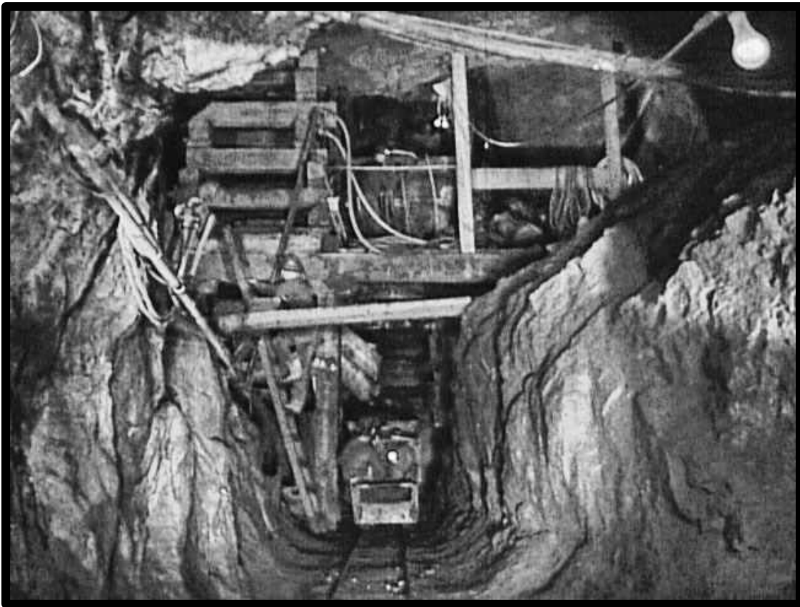
Chute underneath a Cut & Fill Stope, Campbell Mine, c-1940
