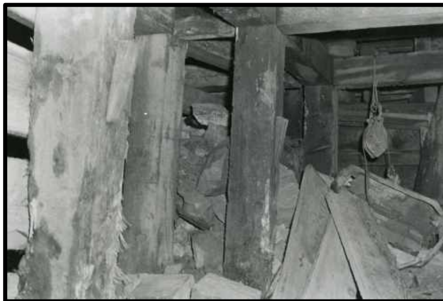
A view of the side of the area Sandoval was killed. His hard hat can be seen in the center of the picture partially covered by a small rock. One of the booms can be seen immediately behind the hat
