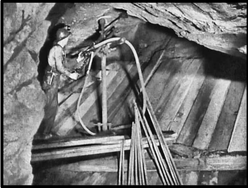
Drilling in an Incline Cut & Fill Stope, Campbell Mine, c-1940
