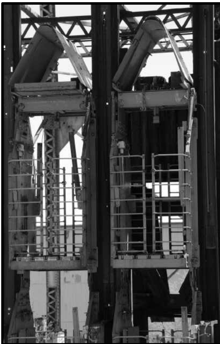
A view of the upper deck on a pair of double deck cages at the Shattuck Mine.
