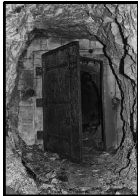
Fire door on the 6 th level station of the Sunrise Shaft.
