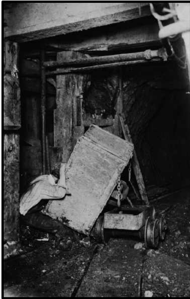
A reenacted safety photo showing a mine car tub that has fallen backwards from a cotter key failure. C-1917
