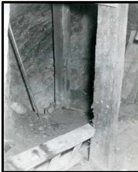
S. Lucero Accident site. 78 Stope, 1400 level Cole Mine
