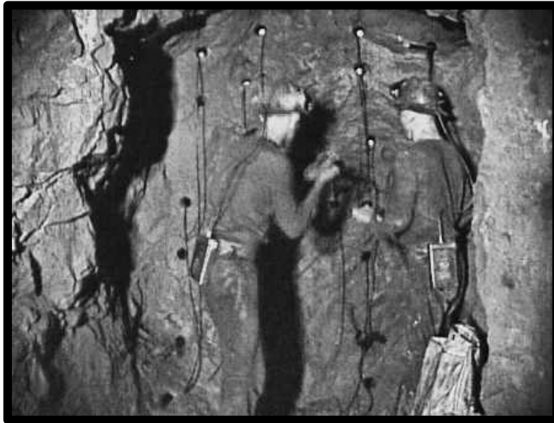
Loading blasting holes in the Campbell Mine C-1938
