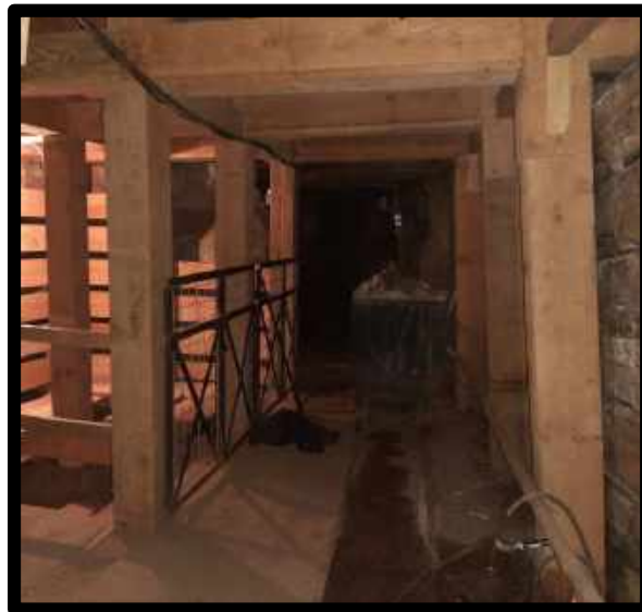
The freshly retimber 3 rd SW Station of the Copper Queen Mine
