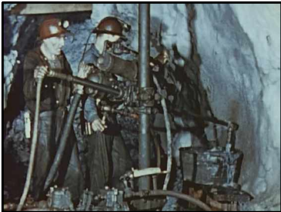
Diamond Drilling in the Campbell Mine C.-1948
