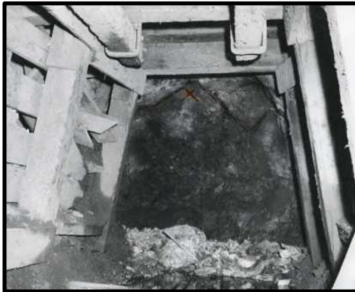
The D.L. Shuck accident site. The original location of the fallen rock is marked in ink on the original image. 22 crosscut 2966 level Campbell Mine.
