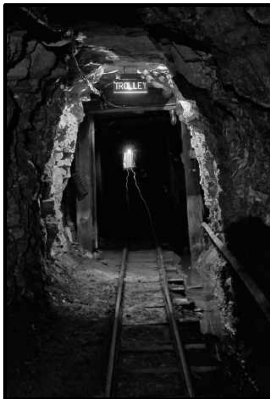
The electrically lit, Queen Tunnel. This amount of illumination is about the same amount Mukovac would have had during his walk from the Lowell to the Gardner Shaft.
