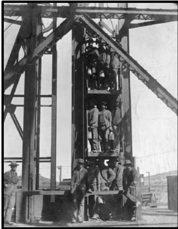
Men being lowered on open cages at the Gardner Mine. C-1909
