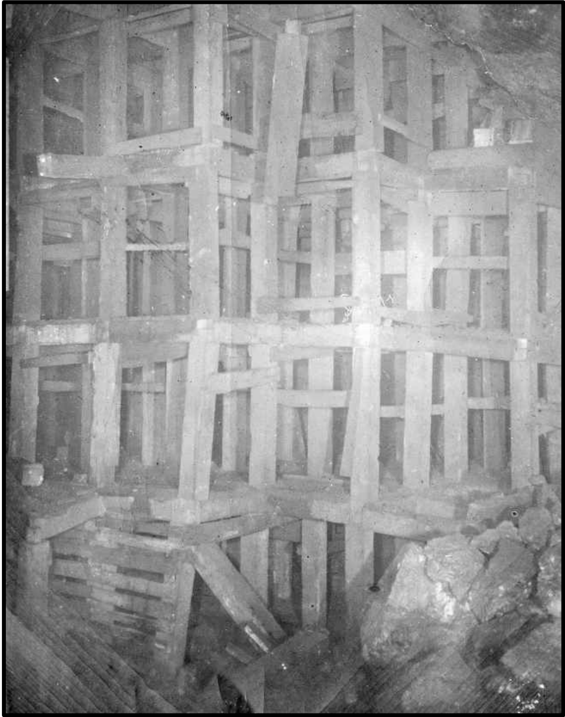
A square-set stope that has not been backfilled, c-1905
