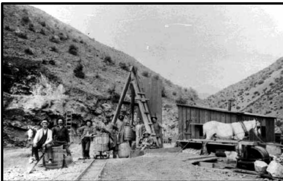
Cochise Mine c-1901. The shaft has a simple “Montana” style headframe. A horse whim is used for hoisting
