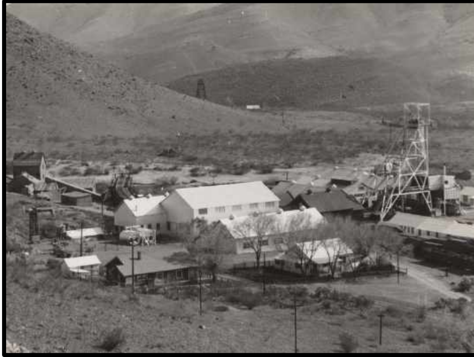
The Denn Mine with the headframe of the Saginaw Shaft in the background.
