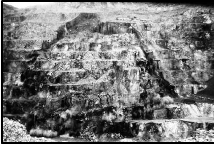
The wall failure in the Holbrook Extension as it was falling in 1970
