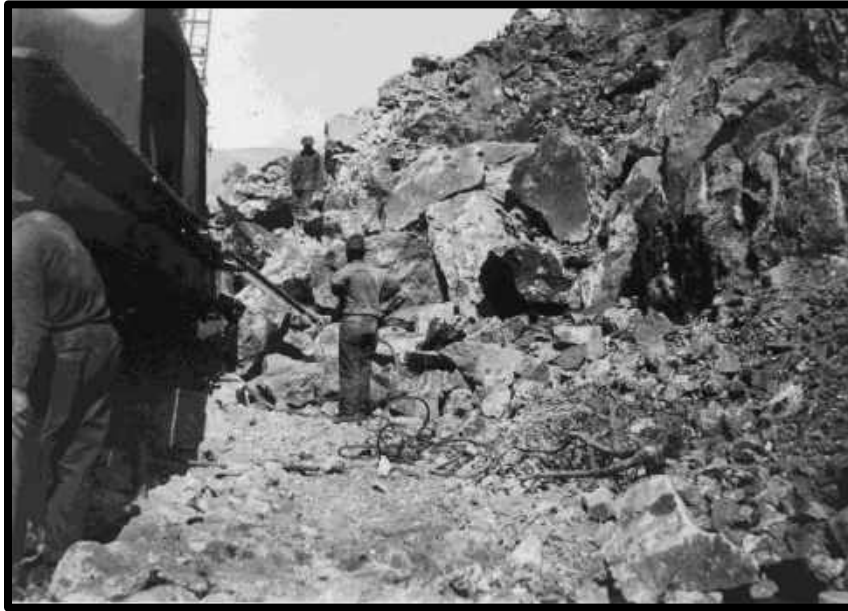
Boulders near a steam shovel jack arm
