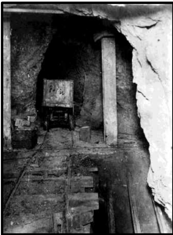
Above: A safety photo showing an open raise (foreground right)
