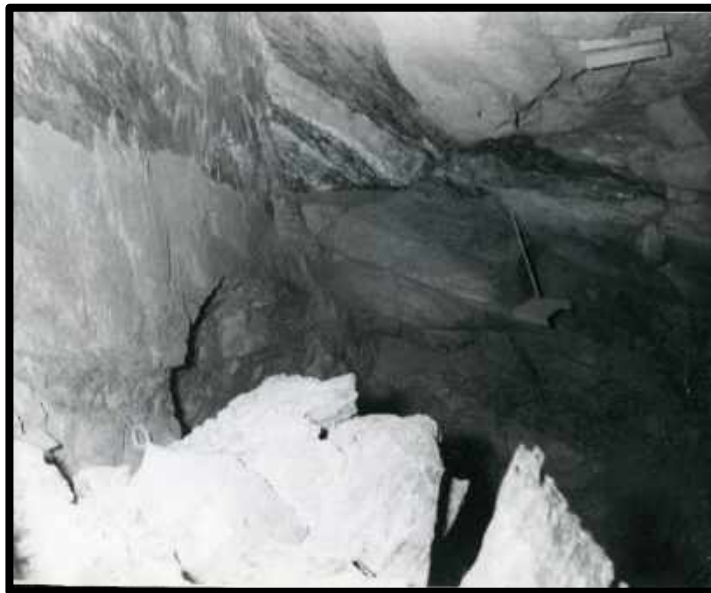
Accident site of F. Duarte, 167-A stope 1300 level Cole Mine
