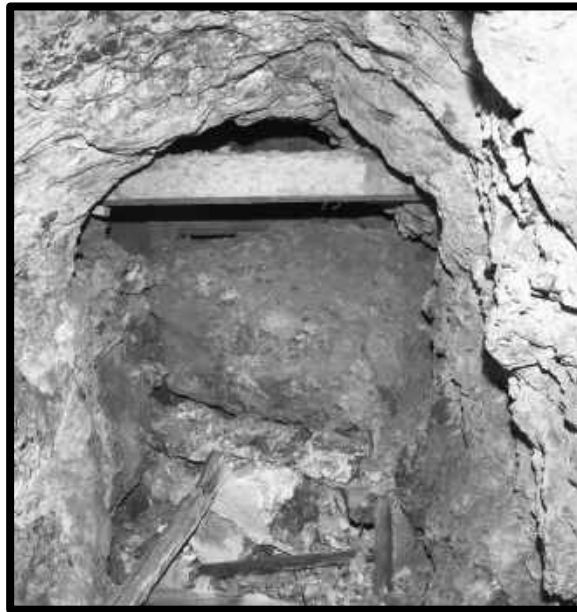
Fallen slab in No. 30 crosscut, 5th level Southwest Mine.
