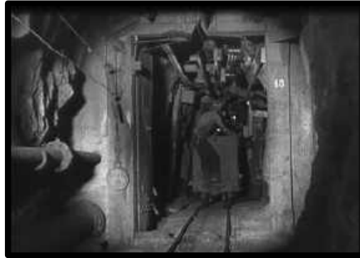
A train passing through the same air door as in previous image.
