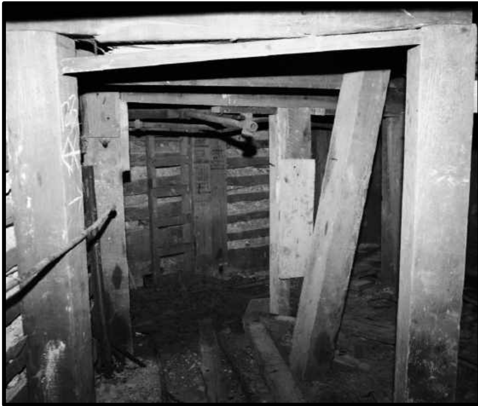
1 st level station of the Hargis Incline.
