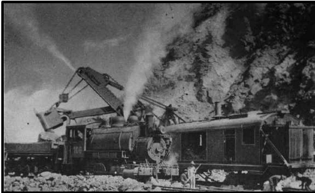
A steam locomotive and steam shovel in the Sacramento pit.
