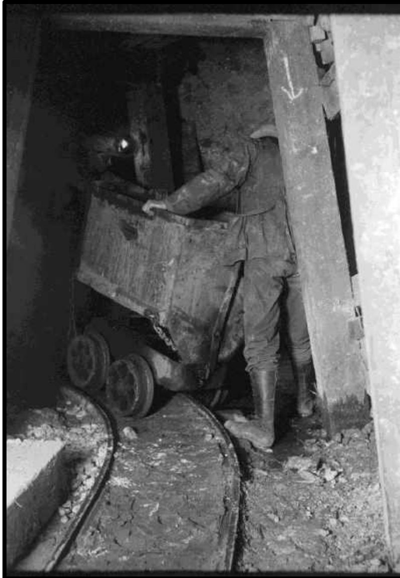
A safety photo showing a miner about to be caught between a mine car and a timber. C-1917
