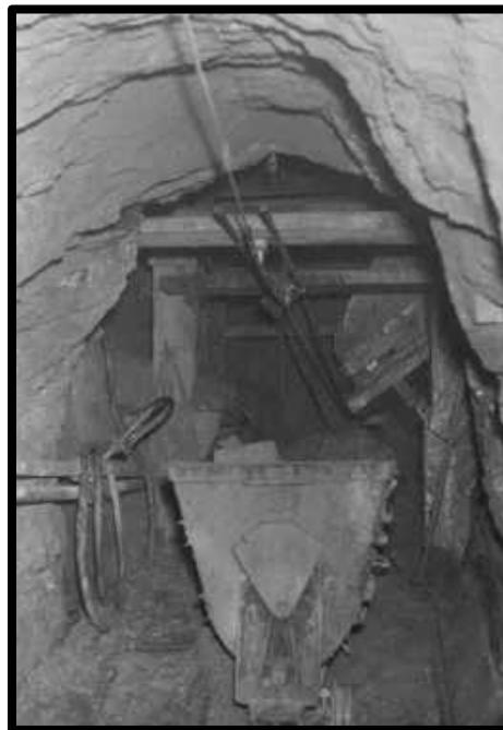
Two views of the V. Rodriguez accident at 129 gen chute on the 1100 level Cole Mine. Note the crosscut has been largely sealed by flowing mud
