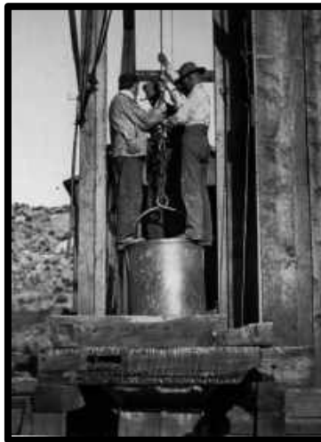
Men riding a sinking bucket at the Dallas Shaft. C-1911
