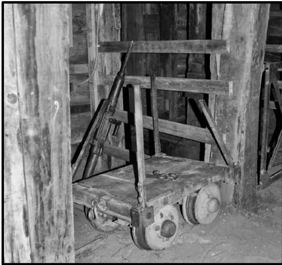
Timber truck at the 3 rd Southwest station of the Copper Queen Incline Shaft
