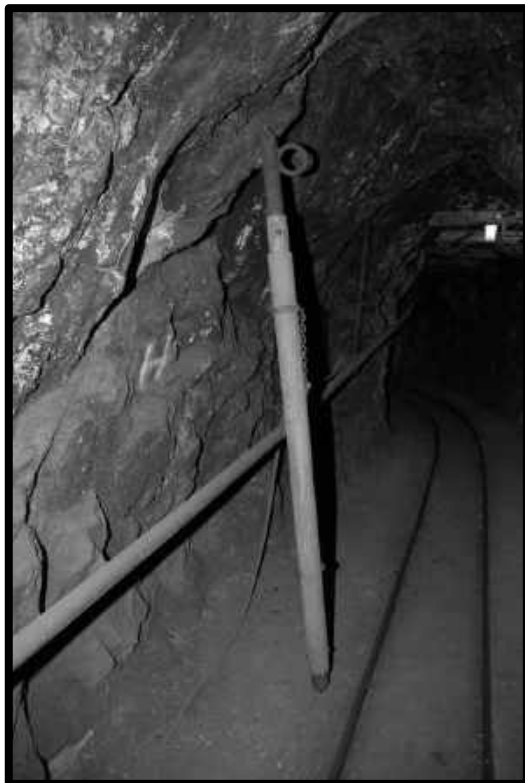
A gin pole resting on the rib of the main drift, 3 rd level Southwest Mine.
