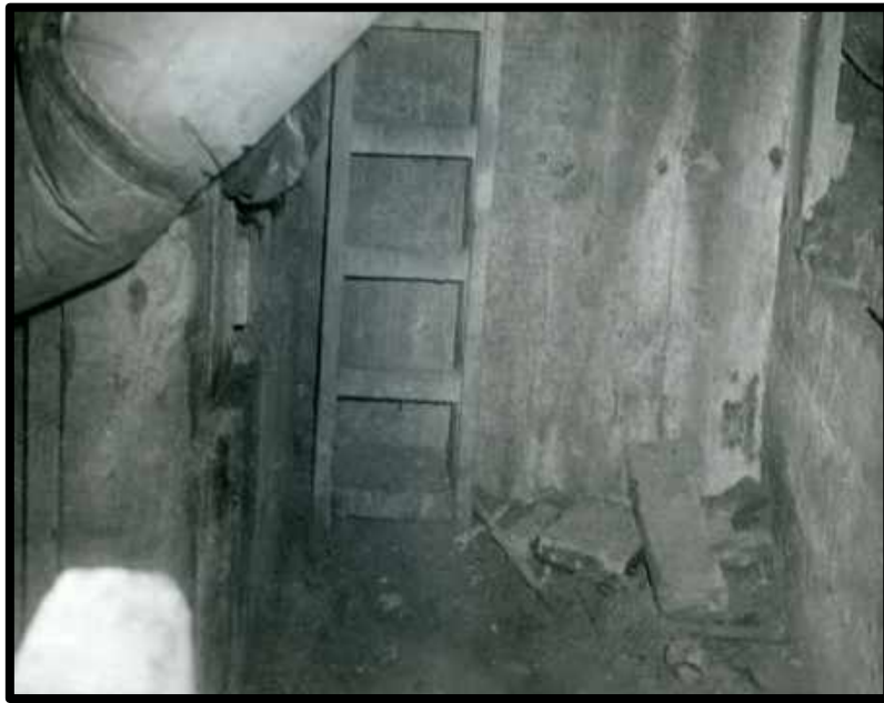
Manway in 24-A stope on the 1650 level of the Dallas Mine. J.E. Cordova accident site
