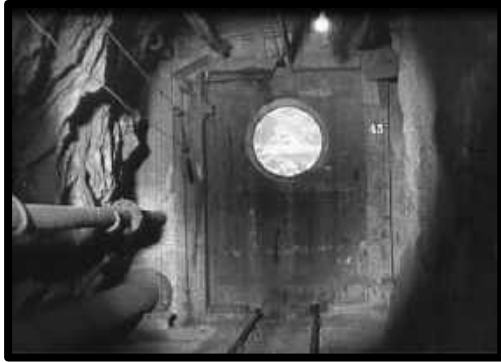
An air door in the Campbell Mine. The round circle is called a target and was applied to make the door easier to see. (left image)
