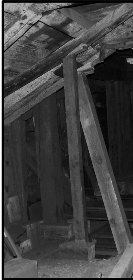
TEMPORARY STULL (s) Two TEMPORARY STULLS SUPPORTING SEGMENT SETS AT THE 3 RD LEVEL SOUTHWEST SHAFT STATION
