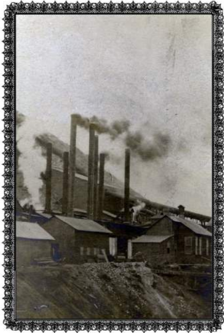
The Copper Queen Smelter c-1902
