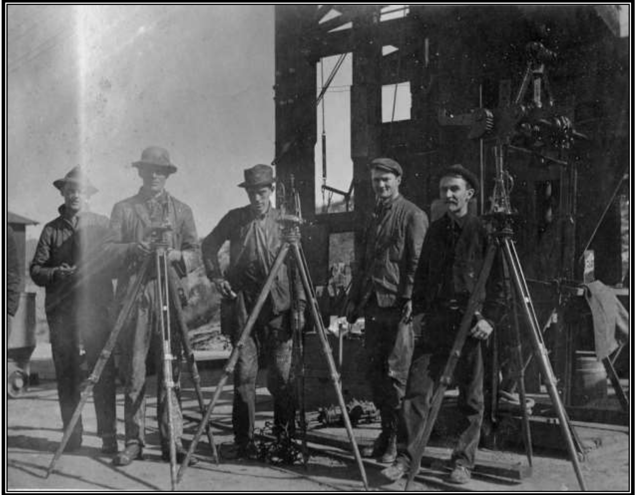
Underground survey crews at the Lowell Shaft - 1904
