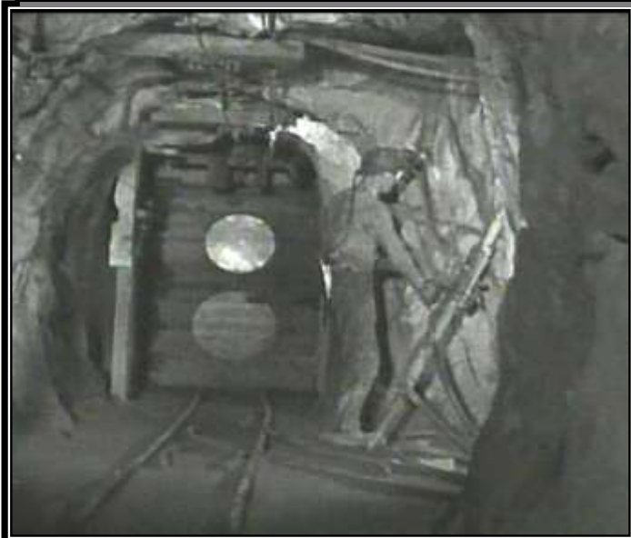
GRAEME LARKIN COLLECTION 65,000 CUBIC FOOT/ MINUTE FAN, 2200 LEVEL CAMPBELL MINE -1939
