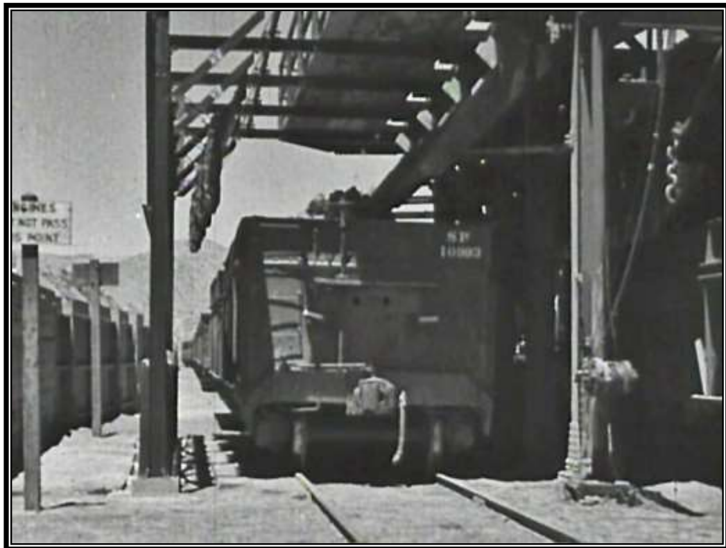
Loading railcars from the ore bin at the Campbell Shaft -1939 Graeme Larkin collection
