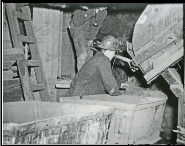
Left: Preparing to start loading “H” cars from what appears to be a new “Verde” style chute in the Campbell Mine C-1955.
