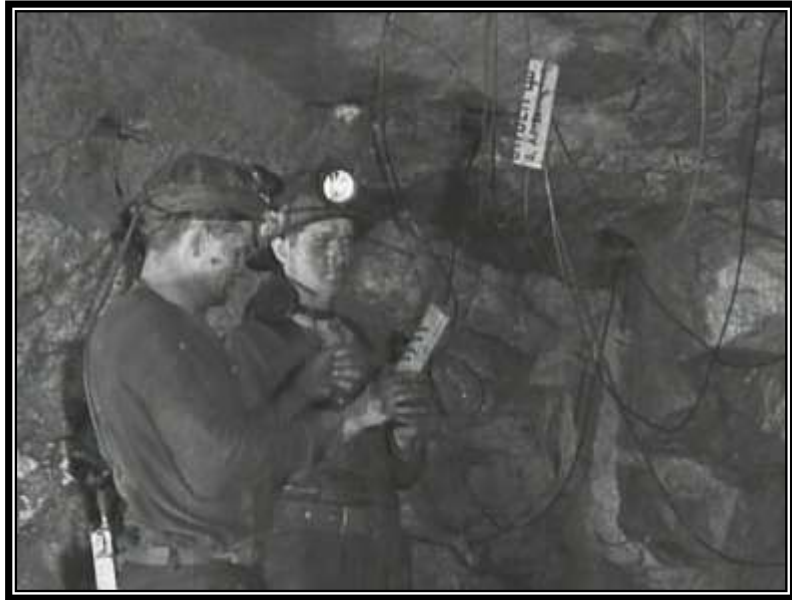
Placing fuses in a spitter board – 1939. Note: the spitter boards are made from Apache Powder boxes. Graeme Larkin collection
