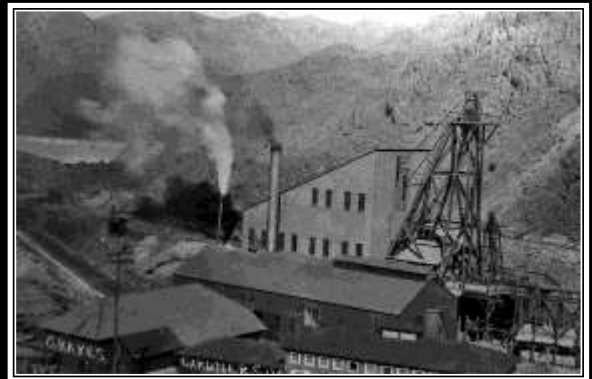
GARDNER SHAFT COMPLEX — OPEN HEAD FRAME, HOIST HOUSE AND SHOPS C-1906.
