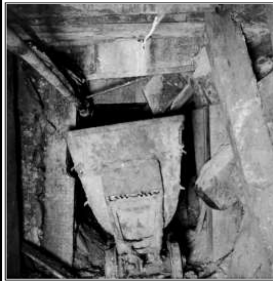
GRAEME LARKIN COLLECTION HEAVILY TIMBERED AREA DISTORTED BY PRESSURE— 1915
