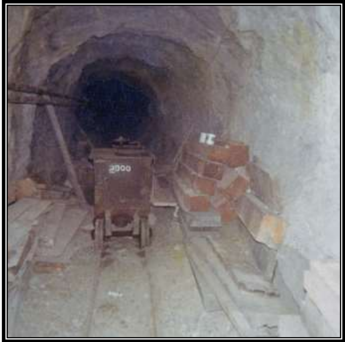
Toilet car on the 2966 level of the Campbell Mine 1970. The setting is typical - a little used, dry crosscut near the working stopes.
