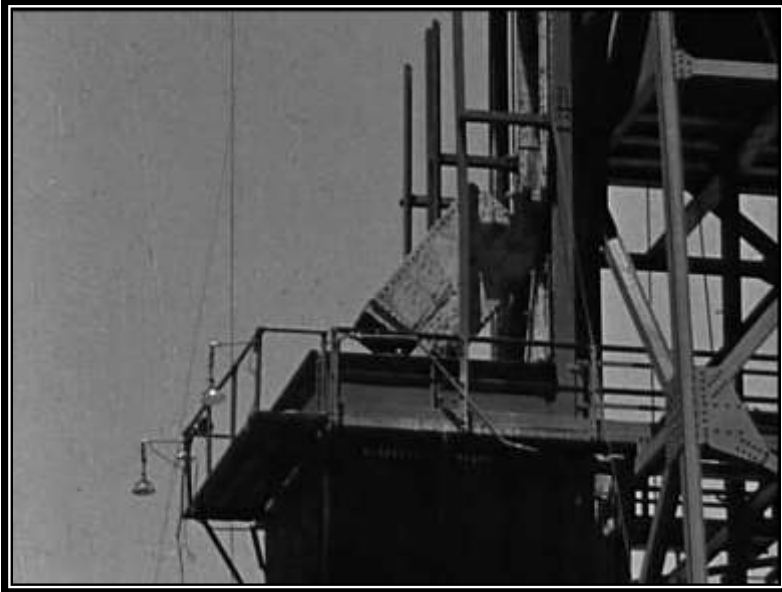
Skip dumping into the ore bin at the Campbell Shaft -1939 Graeme Larkin collection
