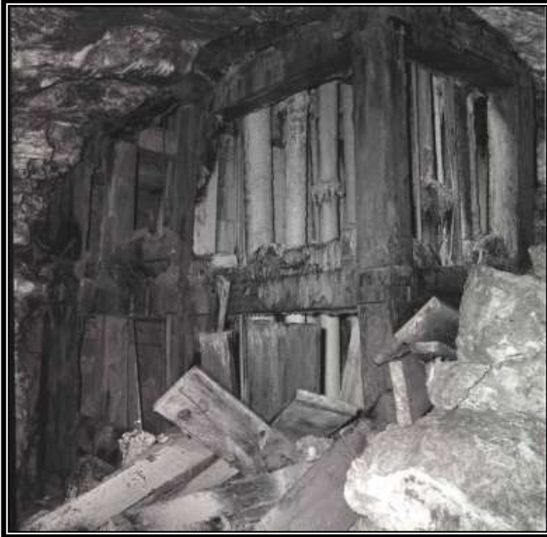
Collapse of the 400 level Czar Mine station due to a lack of timber maintenance - 1964 Graeme Larkin collection
