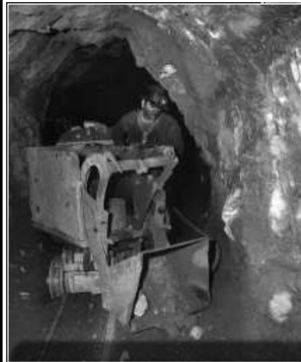
EIMCO OVERSHOT LOADER WORKING IN A CROSSCUT IN THE CAMPBELL MINE - 1939 (R) GRAEME LARKIN COLLECTION
