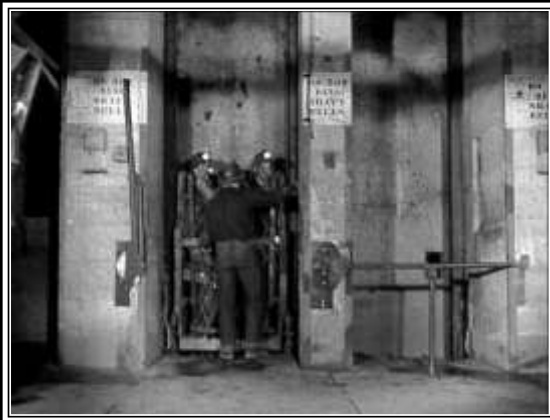
GRAEME LARKIN COLLECTION CAGER ABOUT TO PULL THE SHAFT BELL TO SIGNAL THE HOIST ENGINEER TO STOP THE CAGE, CAMPBELL MINE - 1939
