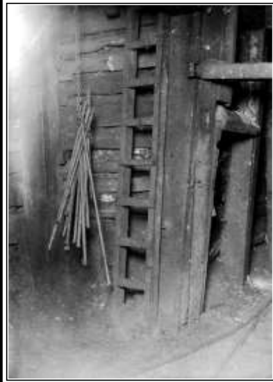
GRAEME LARKIN COLLECTION SAFETY PHOTO SHOWING THE WRONG WAY TO HOIST DRILL STEEL INTO A STOPE C - 1915
