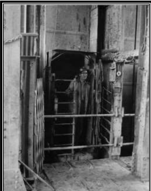
Cager at surface (L), Campbell mine -1974 Pete Kresan photo
