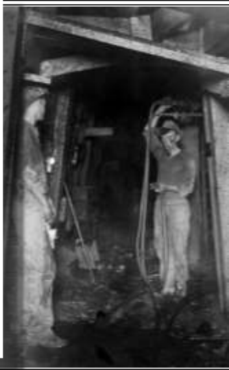
GRAEME LARKIN COLLECTION MEN USING STOPE LAMPS IN A STOPE C - 1915
