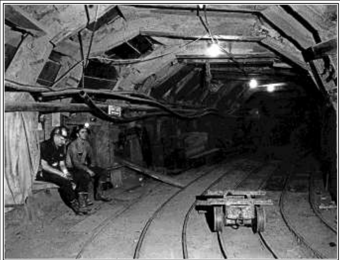
GRAEME LARKIN COLLECTION ENGINEERS WITH WHEAT MARK II LAMPS WAITING FOR THE CAGE, 2700 LEVEL STATION , CAMPBELL MINE - 1974
