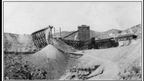
SPRAY SHAFT COMPLEX WITH ENCLOSED HEAD FRAME/HOIST HOUSE, ORE BINS, AND ROCK WASTE AREA C-1905.
