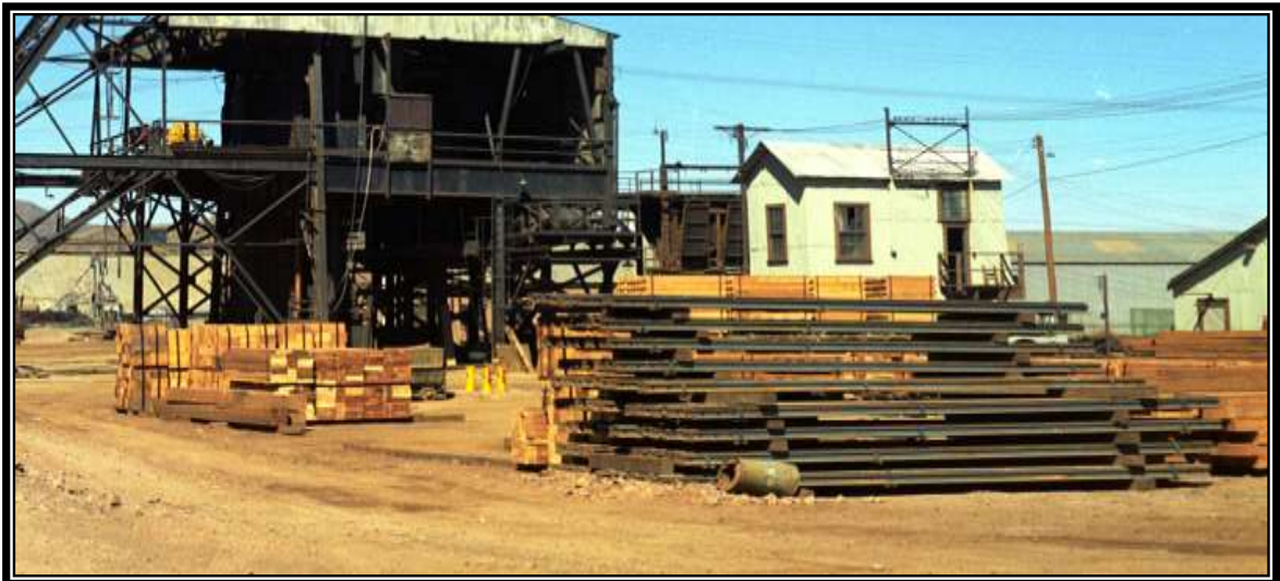
Supplies in steel-banded bundles at the Junction mine yard ready to be lowered into the mine – 1962 Graeme Larkin collection
