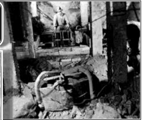
COMPRESSED AIR SLUSHER MOVING BROKEN ROCK IN A STOPE 1938 (R) BISBEE MINING & HISTORICAL MUSEUM COLLECTION
