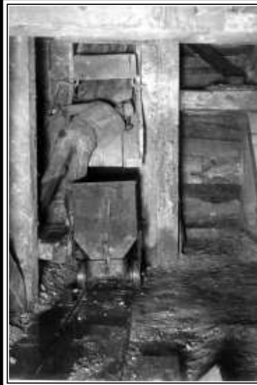
GRAEME LARKIN COLLECTION CLEARING A HUNG CHUTE C - 1915
