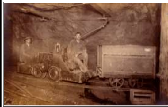
GRAEME LARKIN COLLECTION 2 1/2 TON MOTOR HAULING "GABLE BOTTOM" STYLE CARS, C - 1910
