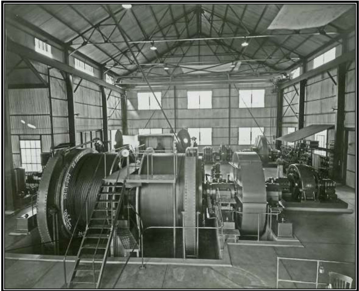
The large Allis Chalmers, grooved drum hoist for the number three and four hoisting compartments at the Junction Shaft, soon after instillation was complete 1934.
