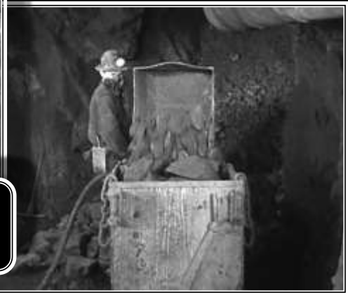
EIMCO OVERSHOT LOADER WORKING IN A CROSSCUT IN THE CAMPBELL MINE - 1939 (R) GRAEME LARKIN COLLECTION
