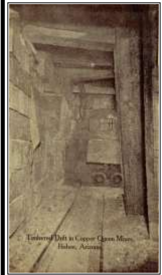
GRAEME LARKIN COLLECTION HEAVY TIMBERING IN A DRIFT — 1910
