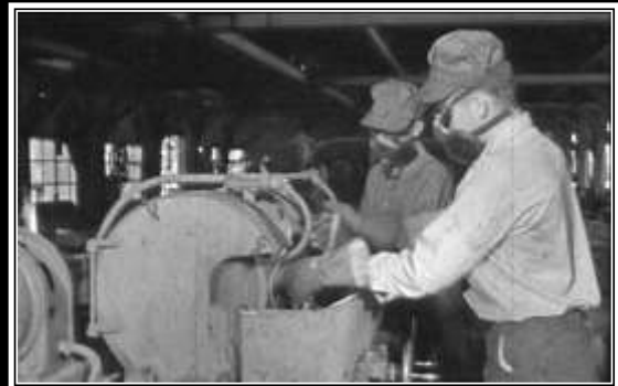
GRAEME LARKIN COLLECTION SHARPENING DETACHABLE DRILL BITS IN BLACKSMITH SHOP - 1939
