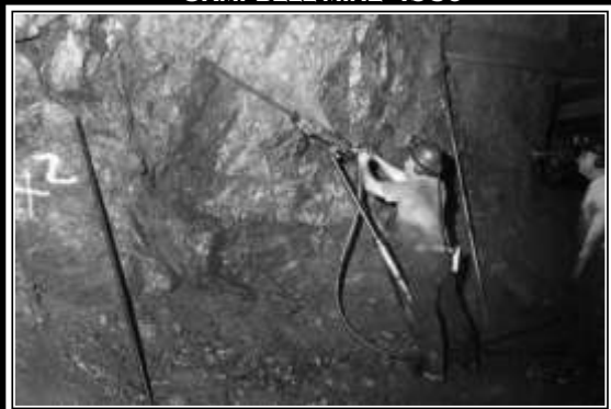
GRAEME LARKIN COLLECTION DRILLING WITH A JACKLEG ON THE 2833 LEVEL CAMPBELL MINE -1973
