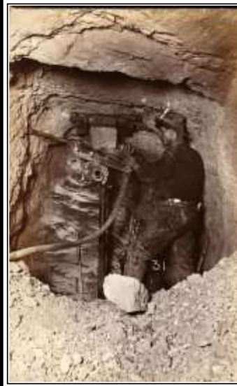
GRAEME LARKIN COLLECTION EARLY BAR AND COLUMN SETUP C - 1908
