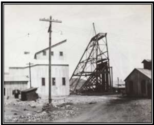
The wooden headframe at the Junction Mine is being overbuilt by a large, steel headframe which will replace it when complete. A new hoist was also added, 1906. Graeme Larkin Collection
