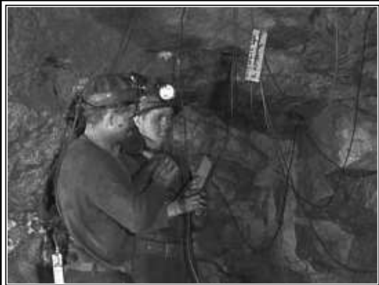
GRAEME LARKIN COLLECTION MINERS USING EARLY EDISON CAP LAMPS, CUTTING FUSES IN A STOPE IN THE CAMPBELL MINE- 1939
