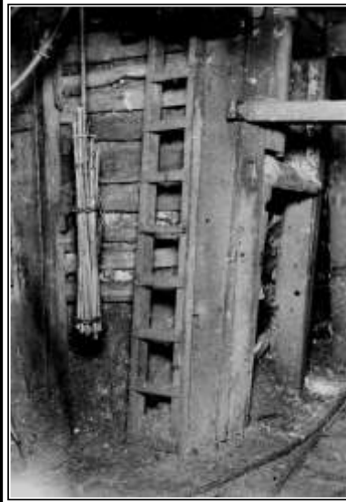
GRAEME LARKIN COLLECTION SAFETY PHOTO SHOWING THE CORRECT WAY TO HOIST DRILL STEEL INTO A STOPE C - 1915
