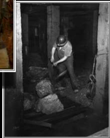
BREAKING BOULDERS ON THE GRIZZLIES IN A CUT AND FILL STOPE 2833 LEVEL CAMPBELL MINE - 1973 GRAEME LARKIN COLLECTION
