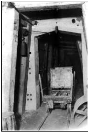
GRAEME LARKIN COLLECTION AUTOMATIC STEEL FIRE DOORS- IN CONCRETE FRAMES C -1915
