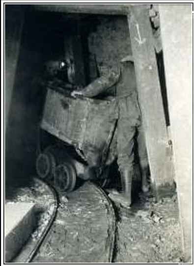
GRAEME LARKIN COLLECTION MEN USING CAP LAMPS RE-RAILING AN “A” STYLE CAR C - 1915
