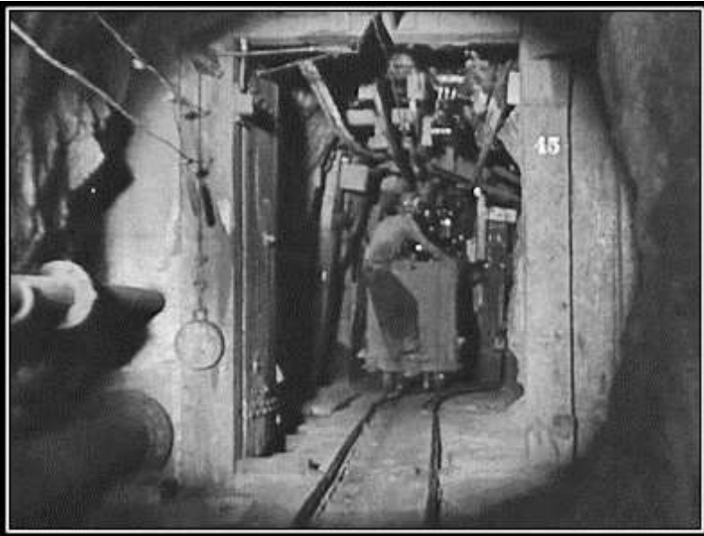
Motor passing through an open air door in the Campbell mine - 1939 Graeme Larkin collection
