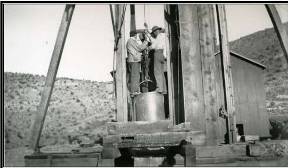
SINKING OF THE COCHISE SHAFT C-1902. NOTE THE TRIPOD HEADFRAME AND THE HORSE WHIM FOR HOISTING OF ROCK. THE MINERS ARE IN WET GEAR TELLING OF WATER AND THE PLANK EXTENSION OF THE HEADFRAME IS TO ENHANCE NATURAL VENTILATION, SUGGESTING A HOT WORK ENVIRONMENT.
