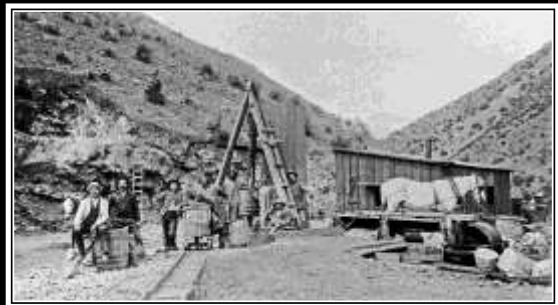
SINKING OF THE COCHISE SHAFT C-1902. NOTE THE TRIPOD HEADFRAME AND THE HORSE WHIM FOR HOISTING OF ROCK. THE MINERS ARE IN WET GEAR TELLING OF WATER AND THE PLANK EXTENSION OF THE HEADFRAME IS TO ENHANCE NATURAL VENTILATION, SUGGESTING A HOT WORK ENVIRONMENT.
