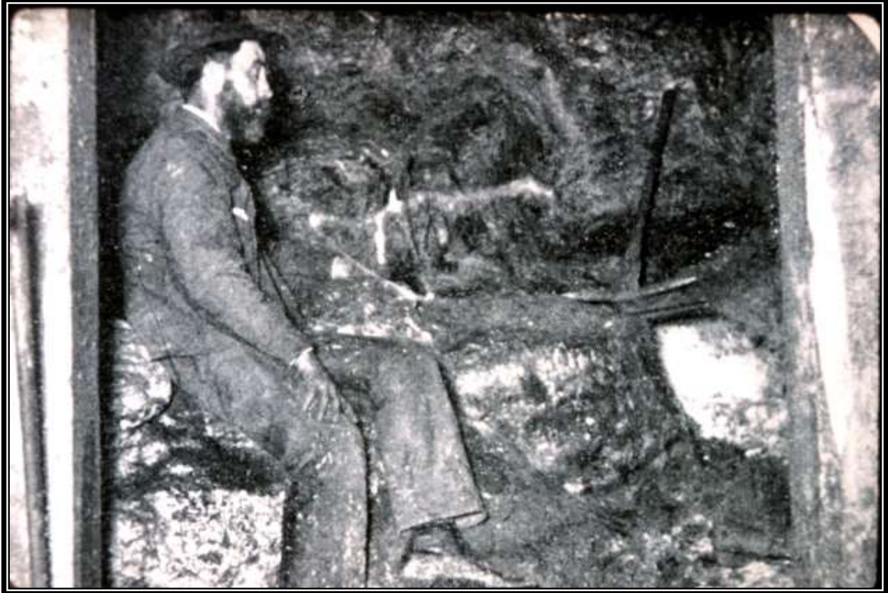
Ben Williams, the first superintendent of the Copper Queen, in the Czar Mine sitting on a ledge formed by the hard ore at the soft ore contact. The material in the upper part of the face could easily be removed by the use of a pick, while the lower would require drilling and blasting. (Douglas, 1900)
