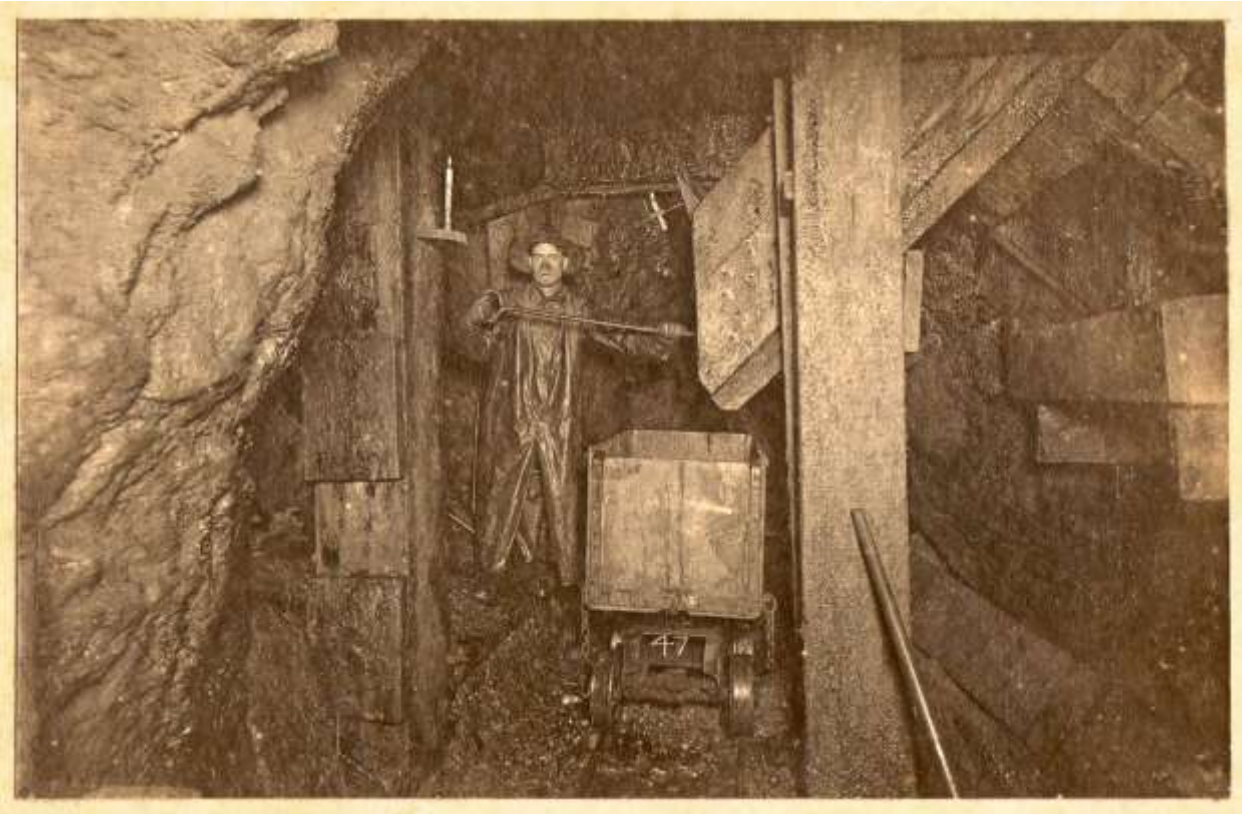
In the above postcard view, the chute door is open, but no muck is coming out. No doubt it was wet (as can be seen) and sticky. His face is mud covered, except where protective goggles (removed for the photograph) were in place. Loading cars in this very common condition was dirty, difficult and very hard work. C - 1910 Graeme Larkin collection
