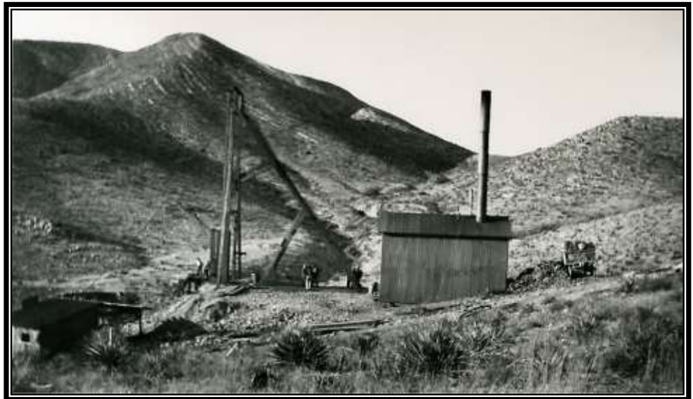
Above: The small wooden head frame at the Dallas Mine as sinking was being initiated C- 1902. Graeme Larkin Collection
