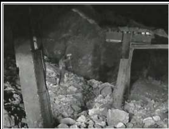
GRAEME LARKIN COLLECTION BREAKING OVERSIZED BOULDERS IN A CUT & FILL STOPE, CAMPBELL MINE -1939
