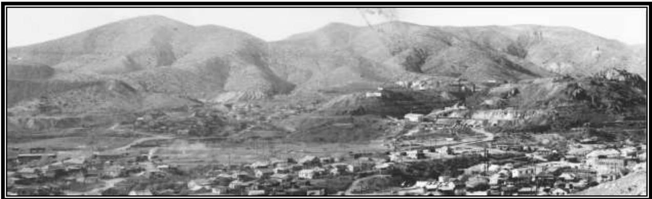
Much the same view of upper Lowell in 1940 with the area that overlay the block caving operations now totally devoid of buildings Graeme Larkin collection
