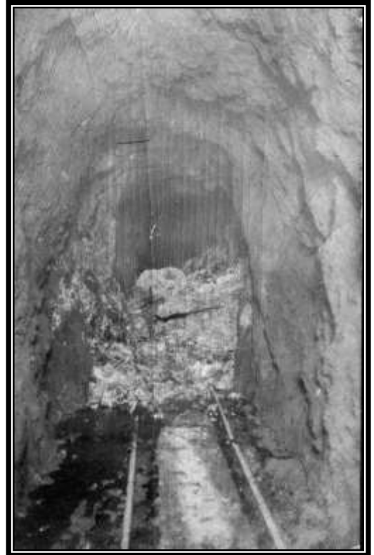
Fall of ground along a fault zone, which should have been an obvious threat and thus timbered - 1904. These are among the most treacherous types of failures as there is often no warning of an impending collapse. Graeme Larkin collection
