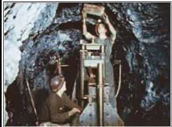
GRAEME LARKIN COLLECTION SETTING UP A DUAL BOOM JUMBO IN THE CAMPBELL MINE -1950
