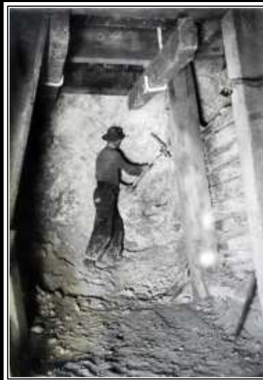
GRAEME LARKIN COLLECTION CLEANING THE FACE UNDER BOOM SUPPORT IN A CROSSCUT C - 1915
