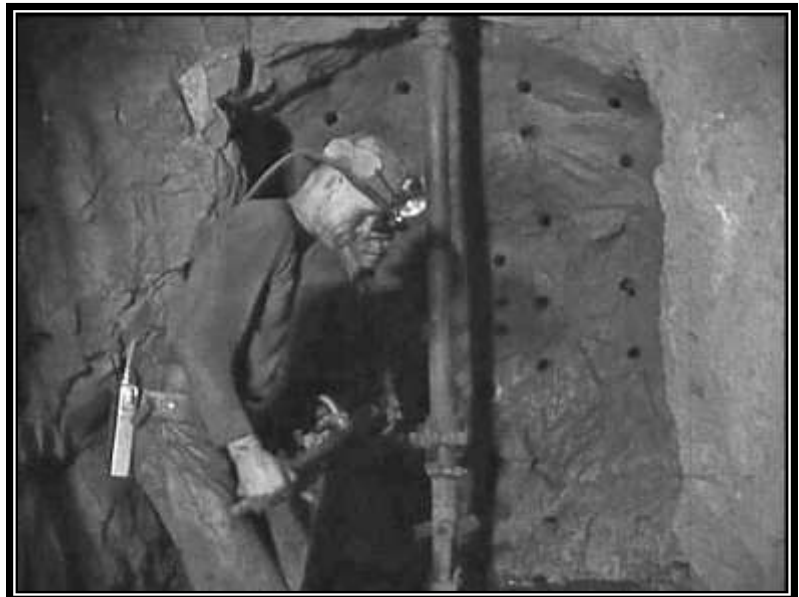
GRAEME LARKIN COLLECTION EARLY BAR AND COLUMN SETUP C - 1908
