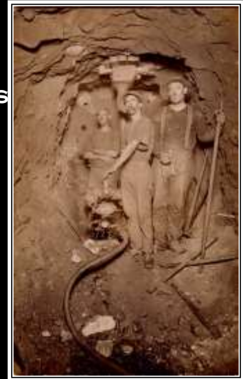
GRAEME LARKIN COLLECTION MINING CREW AT A CROSSCUT FACE DRILLING AND MUCKING C - 1908
