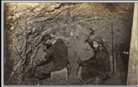
GRAEME LARKIN COLLECTION SINGLE JACK, HAND DRILLING IN A STOPE C - 1903
