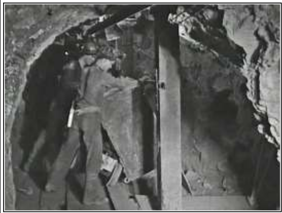
GRAEME LARKIN COLLECTION DUMPING A MINE CAR INTO A RAISE - 1939
