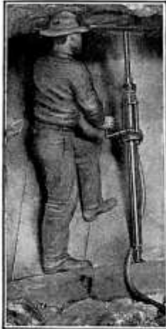
One of the 122 “Waugh” Stopers used by the Copper Queen Consolidated Mining Company of Bisbee, Arizona.
