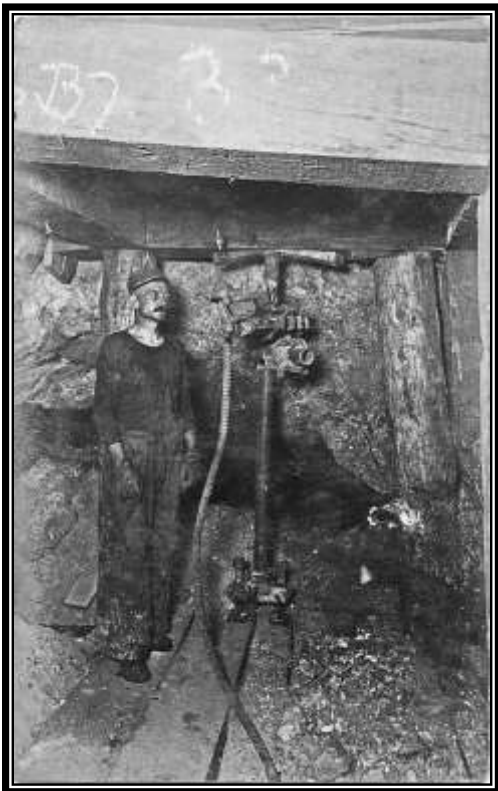
Mining on top of gob in a stope, C - 1910. The hole in front of the drill is the top of the gobbed stope. Graeme Larkin collection
