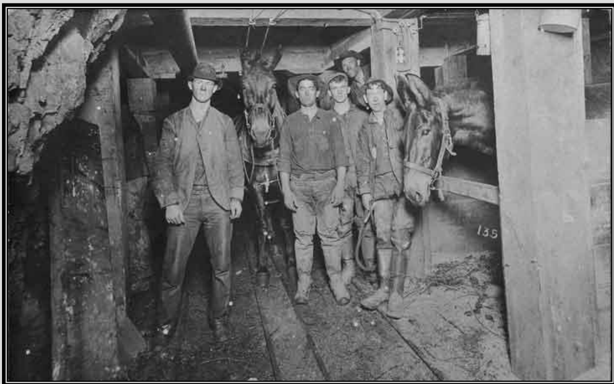
MEN AND MULES UNDERGROUND AT BISBEE, C-1910, THE MUSCLE THAT MINED AND MOVED THE MILLIONS OF TONS OF COPPER ORE WON FROM THE HARD LIMESTONES. THIS PHOTO WAS TAKEN AT MULE BARN IN AN AREA SUPPORTED BY HEAVY, SQUARESET TIMBERING, INDICATING THAT IT WAS AT THE EDGE OF A STOPE. THE MAN AT THE LEFT HAS USED FIRE FUSE AS A BELT, A COMMON, BUT UNWISE PRACTICES. A CANDLESTICK CAN BE SEEN SUSPENDED BY WIRE FROM THE COLLAR OF THE MULE IN THE CENTER, WHILE THE MAN AT THE FAR RIGHT HAS ONE IN HIS HAND AS WELL AS FOUR EXTRA CANDLES IN THE INSIDE POCKET OF HIS JUMPER.
