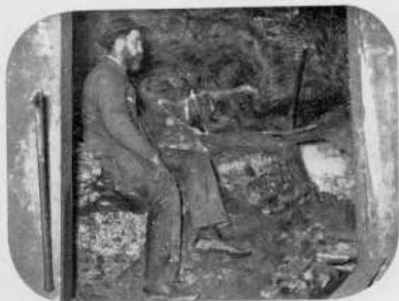
Contorted Clays in the Baxter Tunnel.
