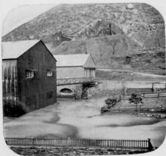
Open-Cut of the Copper Queen Mine.
