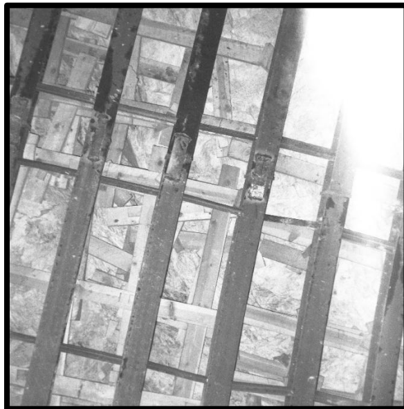
STEEL TIMBERING IN THE BACK OF THE 2966 LEVEL STATION CAMPBELL MINE
