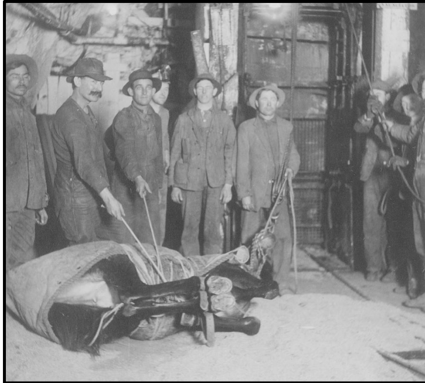
LOADING HARNESS SECURING A MULE THAT HAS BEEN LOWERED UNDERGROUND
