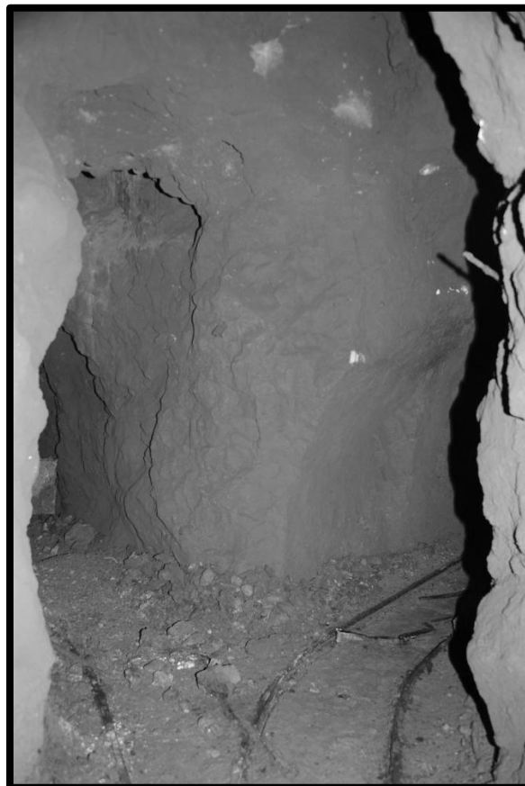
“Y” INTERSECTION 5 TH LEVEL SOUTHWEST MINE
