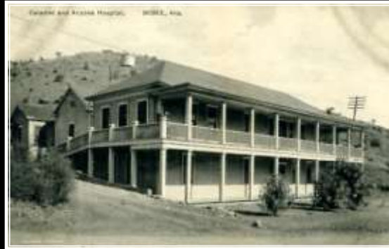
GRAEME LARKIN COLLECTION CALUMET & ARIZONA HOSPITAL NEAR LOWELL C - 1908
