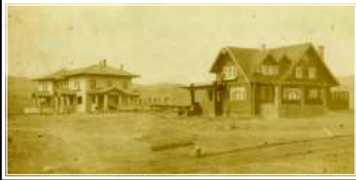
GRAEME LARKIN COLLECTION HOMES BUILT BY THE CQ FOR THE GENERAL MANAGER (L) AND THE CHIEF PHYSICIAN AT THE END OF THE VISTA PARK C - 1910
