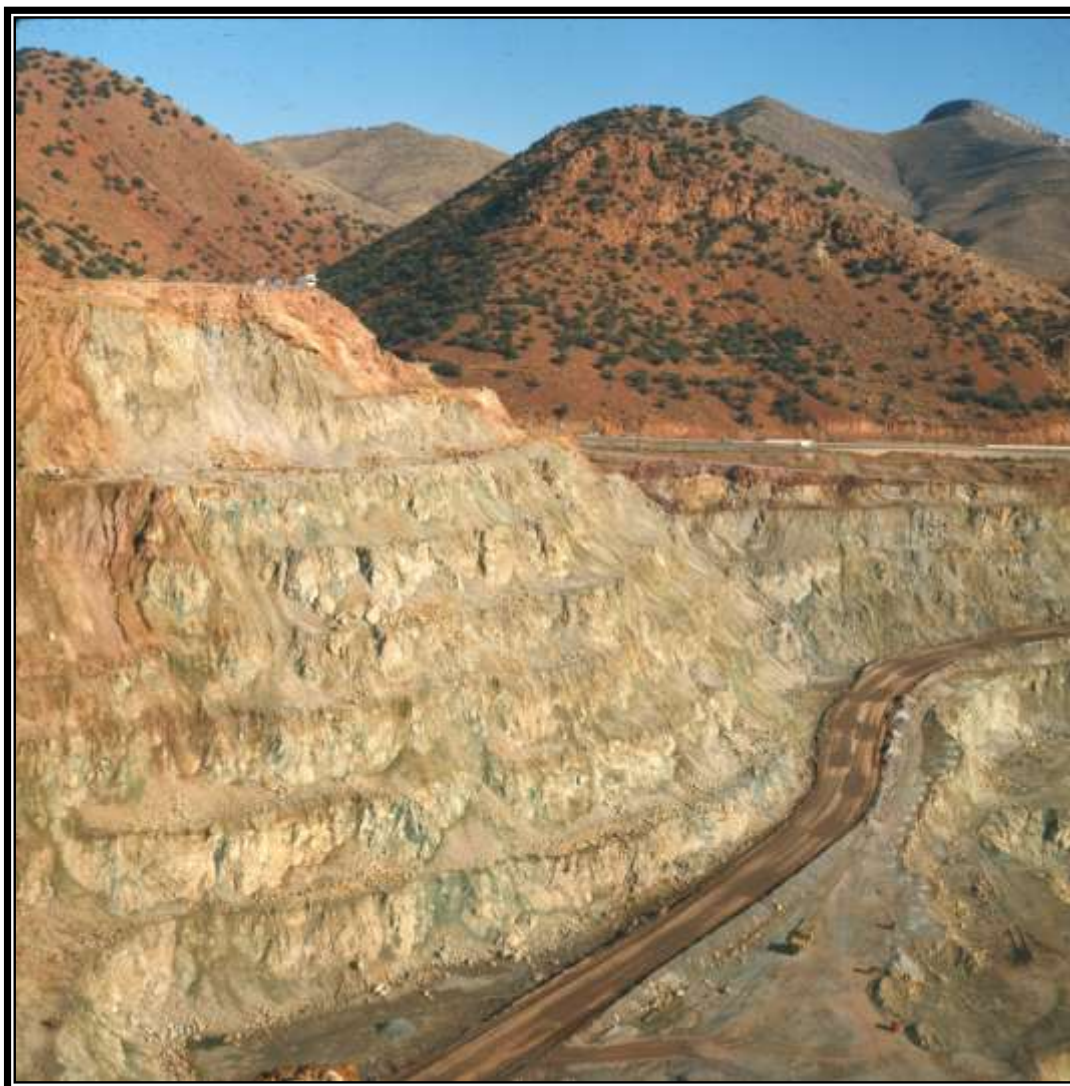
A view of the haul road along the remnant of Sacramento Hill to the primary crusher - 1970. Note that here too, the haul road is well maintained been watered in a manner to minimize erosion of the road surface. This can be seen in the regularly spaced wet areas. Graeme Larkin collection
