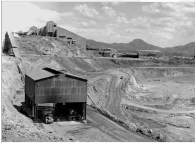
A 35 TON HAUL TRUCK DUMPING ORE DIRECTLY INTO THE PRIMARY CRUSHER, C-1956. GRAEME LARKIN COLLECTION
