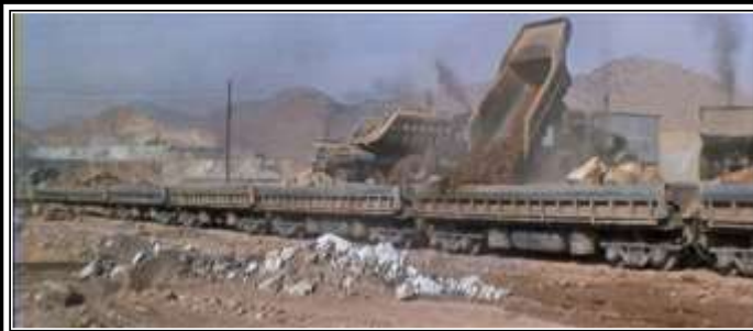
TRANSFERRING NON-MINERAL MATERIAL FROM TRUCKS TO TRAIN FOR TRANSPORT TO THE NUMBER 7 DUMP - 1954. GRAEME LARKIN COLLECTION
