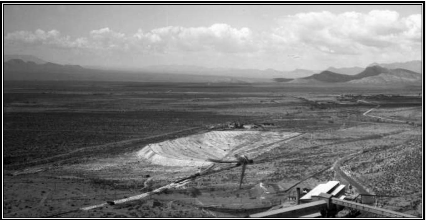
Placement of leach material on the Number 2 dump near Don Luis by train, C -1926. The leach cells on the surface are being developed in preparation for the addition of the leach solutions via the launder along the right side of the dump
