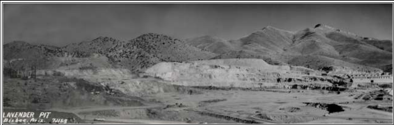
THE LAVENDER PIT IN 1952 , PRESTRIPPING IS WELL ADVANCED WITH THE CONCENTRATOR FOUNDATIONS IN THE RIGHT —CENTER AND THE MAIN PIT SHOP ON THE RIGHT EDGE. A SHOVEL CAN BE SEEN CENTER-LEFT AND BLAST HOLE DRILLS ON THE TOP OF SAC HILL.
