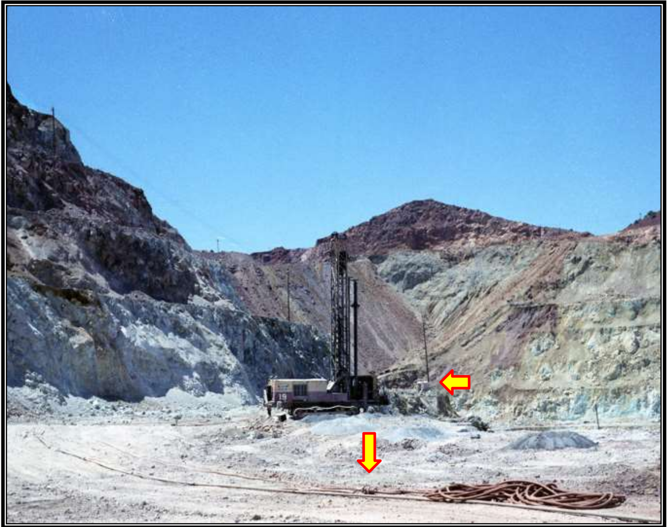
A typical electrical power configuration, with the power line descending along the pit slope and two small switch houses at a drop next to a power pole. A connection of two power cables is in the center foreground and the slack cable is in the lower right foreground – 1965. Graeme Larkin collection
