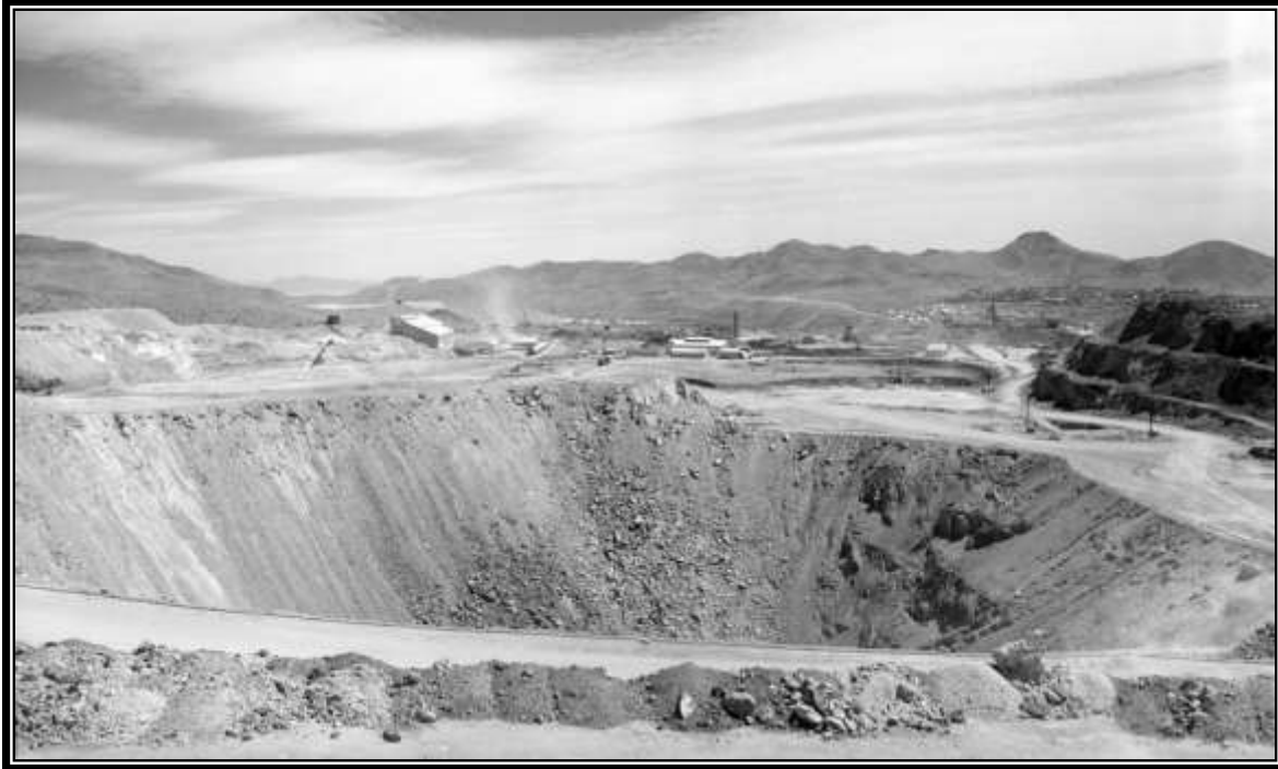
A partially filled Sacramento PIT Mine – 1953. The blocky material on the left was from Sac Hill, while that on the right is overburden from near the Junction. Graeme Larkin collection
