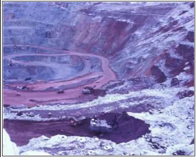
THREE SHOVELS WORKING IN NON-MINERAL MATERIAL ON THE EAST WALL OF THE PIT - 1972. GRAEME LARKIN COLLECTION
