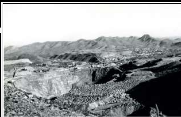
EARLY NON-ORE MATERIAL WAS USED TO BACKFILL THE SAC PIT - 1951. GRAEME LARKIN COLLECTION
