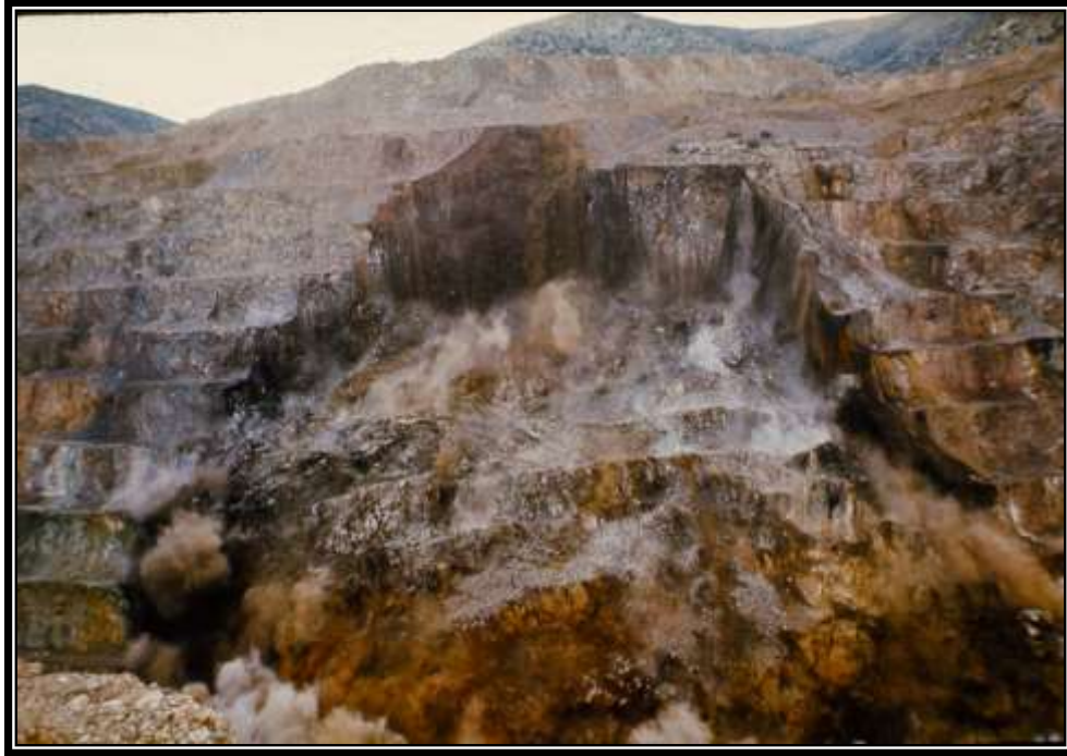
Slope failure of an estimated 300,000 cubic yards in process of full failure in the Holbrook Extension - 1970. Graeme Larkin collection
