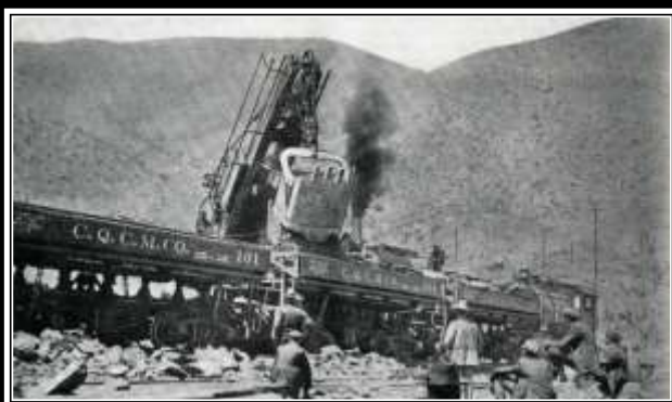
LOCAL RESIDENTS WATCH A SHOVEL LOADING CARS WHILE DIGGING A RAIL CUT INTO SAC HILL — 1917 GRAEME LARKIN COLLECTION
