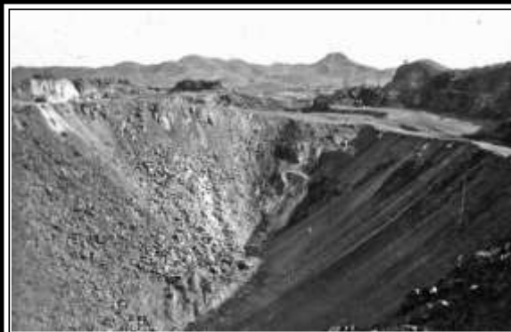
EARLY NON-ORE MATERIAL WAS USED TO BACKFILL THE SAC PIT - 1951. GRAEME LARKIN COLLECTION
