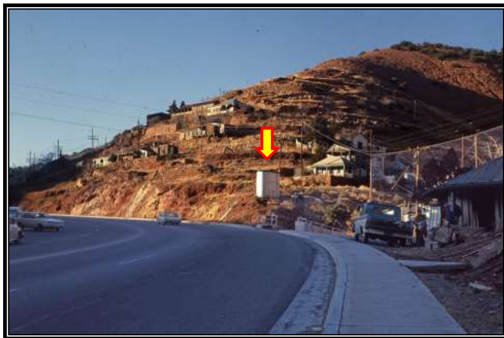
A section of the old Bisbee smelter smoke-stack had been placed over this and one other nearby ventilation shaft, as a safety precaution before 1910. Painted a bright silver-color, in 1963 this one was used for access for most of a year. To the right, men can be seen salvaging lumber from a house that was to be demolished for the pit expansion.
