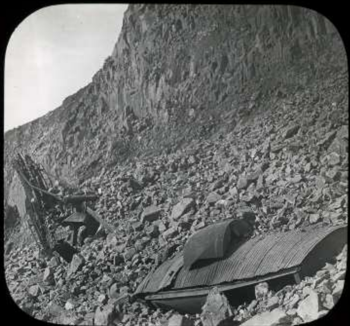
STEAM SHOVEL ALMOST COMPLETELY COVERED BY ROCK CAUSED BY A FAILURE OF THE BENCH FACE, C — 1918. GRAEME LARKIN COLLECTION
