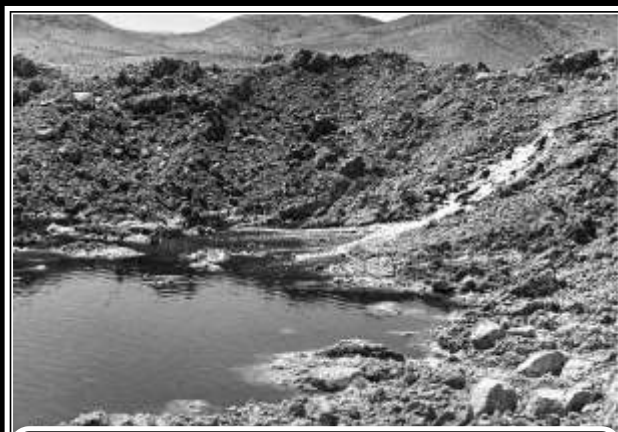
WATER BEING FED INTO A PONDING CELL ON THE TOP OF NUMBER 7 DUMP - 1977 GRAEME LARKIN COLLECTION
