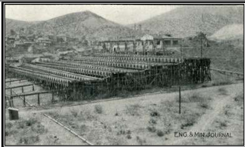
Test facility near the Sacramento Shaft for the development of a precipitation plant to recovery copper from leach material to be produced from the Sacramento Pit -1915 Graeme Larkin collection
