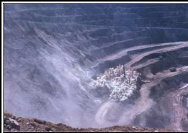
BLASTING THE HOLES SHOWN IN THE PHOTO AT THE LEFT, 1970. NOTE THE DIFFERENT COLOR DUST COLUMNS — LIGHT COLOR ORE, DARK WASTE. GRAEME LARKIN COLLECTION
