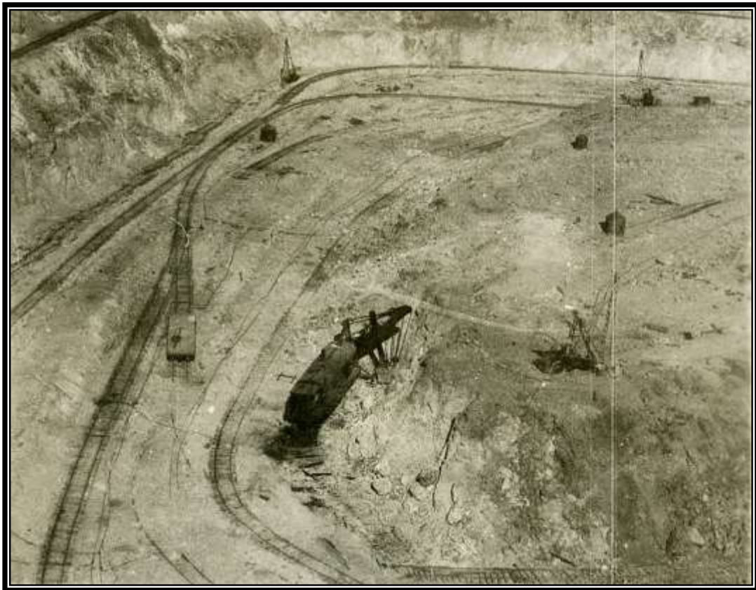
Sacramento Pit C-1928. Note the boulders behind the shovel and the hard toes protruding into the digging pit
