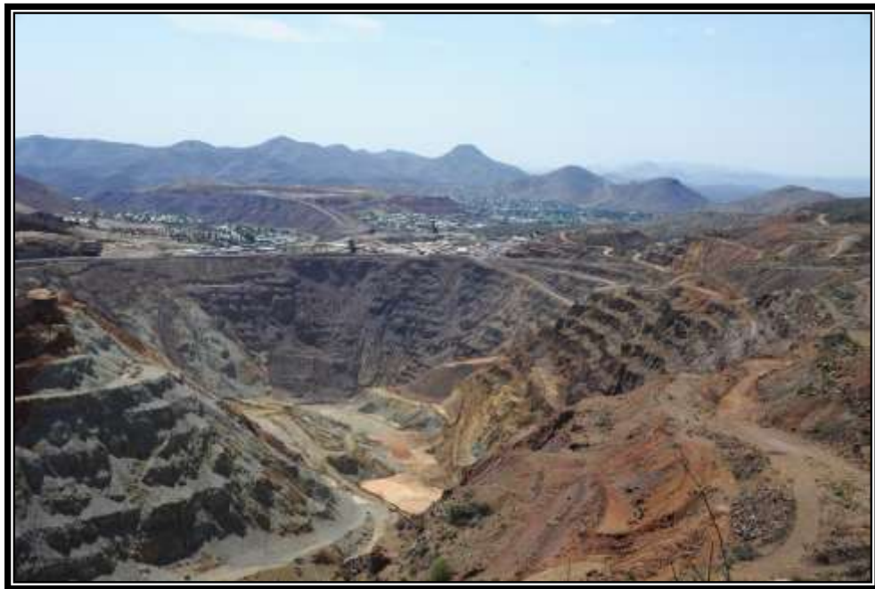
A contemporary view of the east wall of the pit in which the slope failure in the relatively weak Glance Conglomerate can be seen. While this failure began during operations, it caused few problems, although catchment berms were constructed as a precaution.
