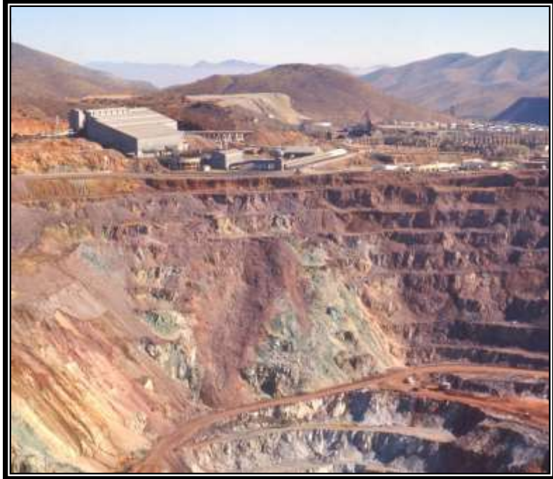
The northeast wall of the Lavender Pit in 1965 with the bulge of the failing pit wall quite obvious. Also apparent is the red/brown material dumped over the slope in 1962 in a futile attempt to slow the movement, as it was causing the highway above to subside a bit.
