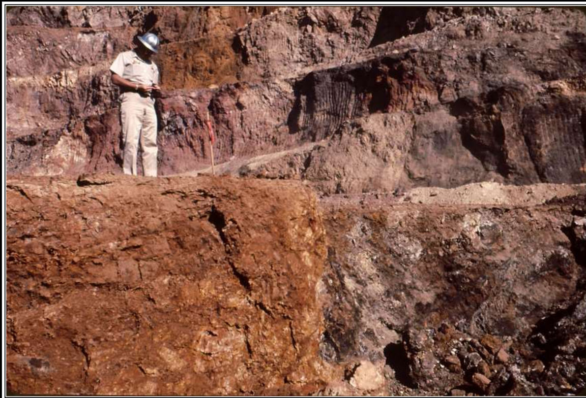
CONTACT BETWEEN OXIDE ORE (LEFT) / LIMESTONE (RIGHT), HOLBROOK EXTENSION – 1970 GRAEME LARKIN COLLECTION
