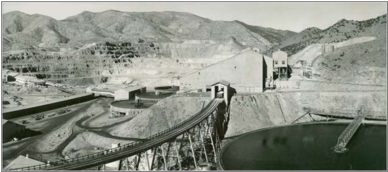
THE LAVENDER PIT AND CONCENTRATOR - 1957 , TAILING THICKENERS IN THE RIGHT FOREGROUND, A RAILCAR OF LIME FROM PAUL SPUR IN THE CENTER AND THE THREE CONCENTRATE THICKENERS CENTER-LEFT. CONCENTRATE DRYING AND LOADING TOOK PLACE IN THE BUILDINGS TO THE LEFT OF THE CON THICKENERS.
