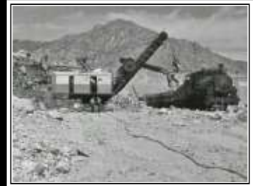
AN ELECTRIC SHOVEL LOADING RAIL CARS IN THE NEW CORNELIA MINE AT AJO C - 1940 GRAEME LARKIN COLLECTION
