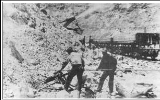
DRILLING TOE HOLES IN THE SAC PIT- 1925 GRAEME LARKIN COLLECTION
