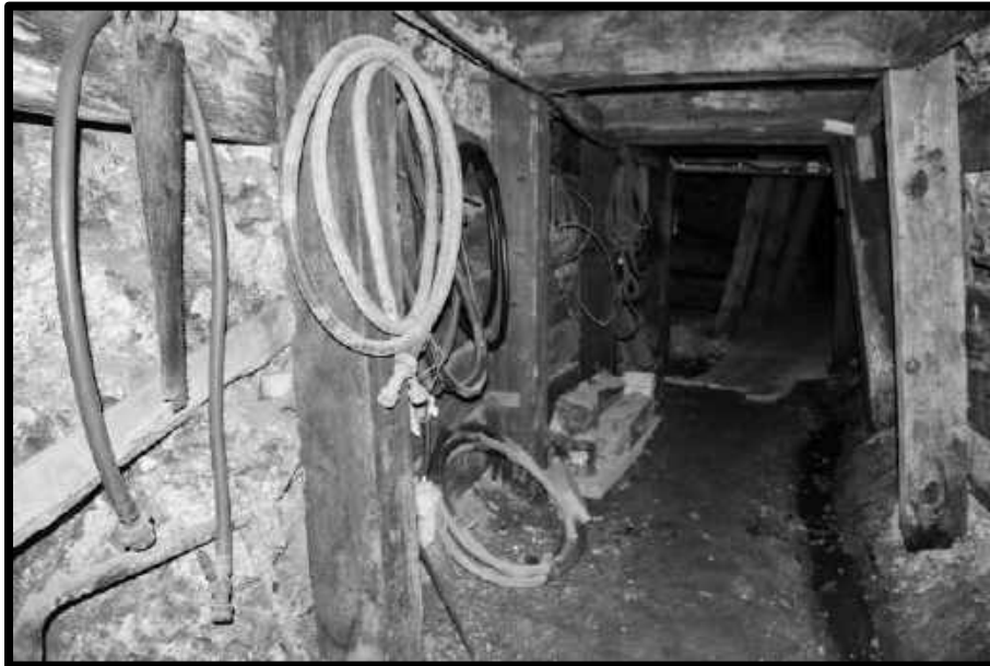
AIR HOSE(S) HANGING FROM THE TIMBER, SOUTHWEST MINE, 3 RD LEVEL, 61 CROSSCUT.
