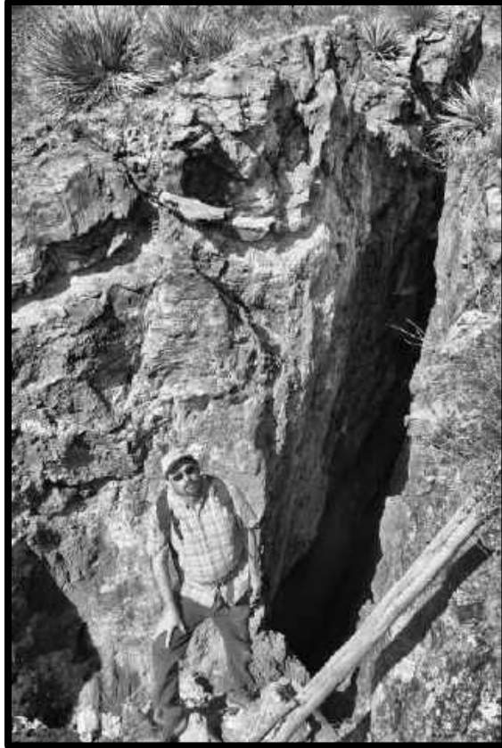
SUBSIDENCE CRACKS ON THE CREST OF QUEEN HILL NEAR THE SUNRISE SHAFT.
