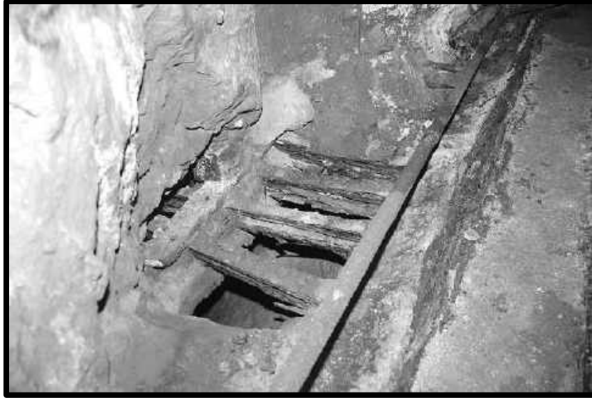
GRIZZLY (ABANDONED) ON 10 RAISE IN 9 CROSSCUT, 6 TH LEVEL SOUTHWEST MINE.
