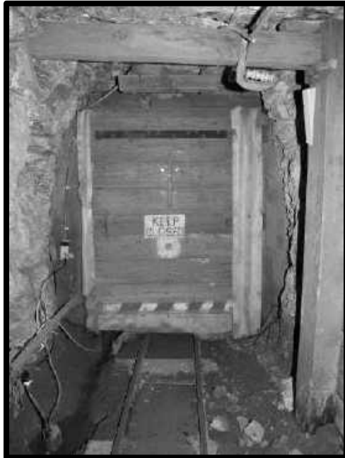
AIR DOOR IN SOUTHWEST MINE, 3 RD LEVEL, 30 CROSSCUT.
