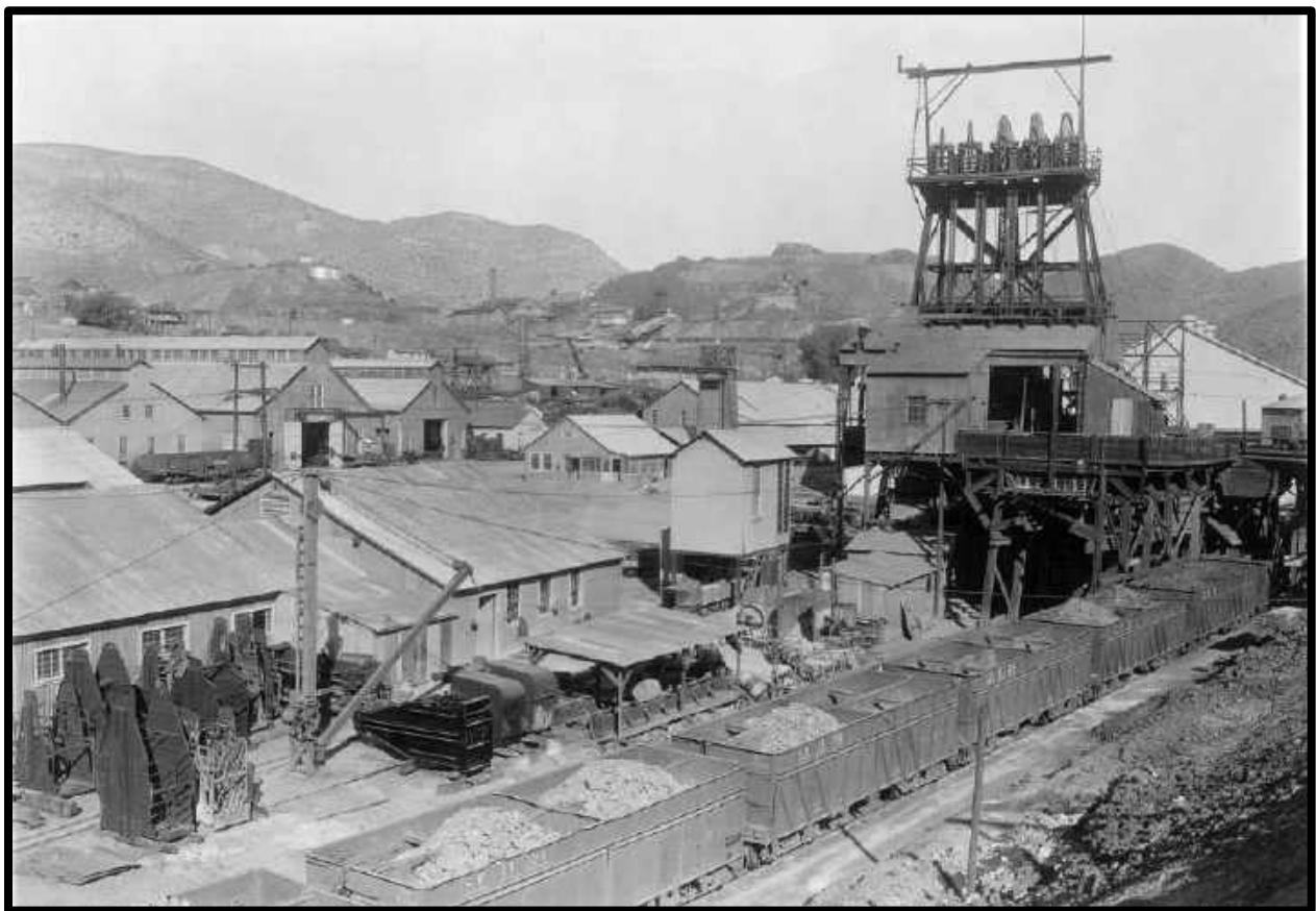
JUNCTION MINE C-1924
