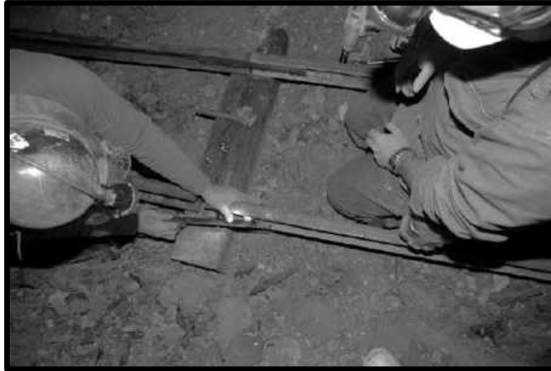
FISH PLATE BEING INSTALLED IN 30 CROSSCUT, 3 RD LEVEL, SOUTHWEST MINE
