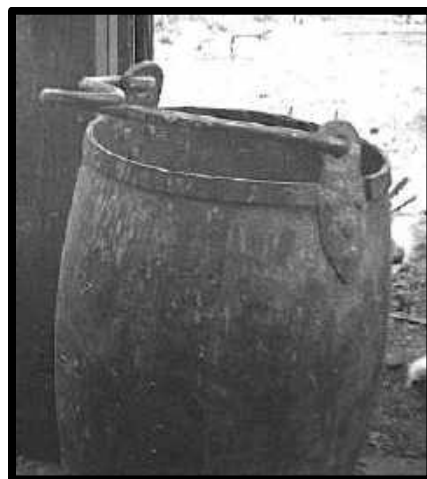
SINKING BUCKET AT THE TOP OF THE DALLAS SHAFT. C-1911
