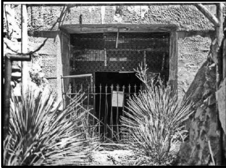
COLE ADIT (ABANDONED)
