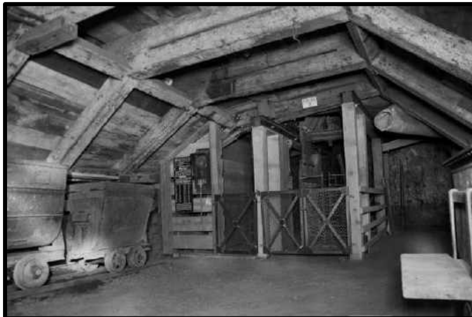
STATION SOUTHWEST SHAFT, 3 RD LEVEL.
