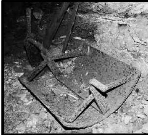
CHUTE DOOR (LOOSE) SOUTHWEST MINE 3 RD LEVEL, 61 CROSSCUT.
