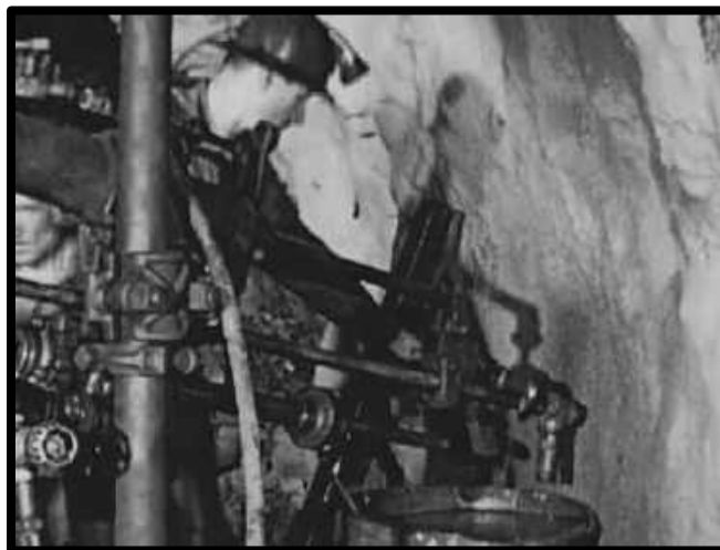
STAND PIPE CAMPBELL/JUNCTION MINE C-1940
