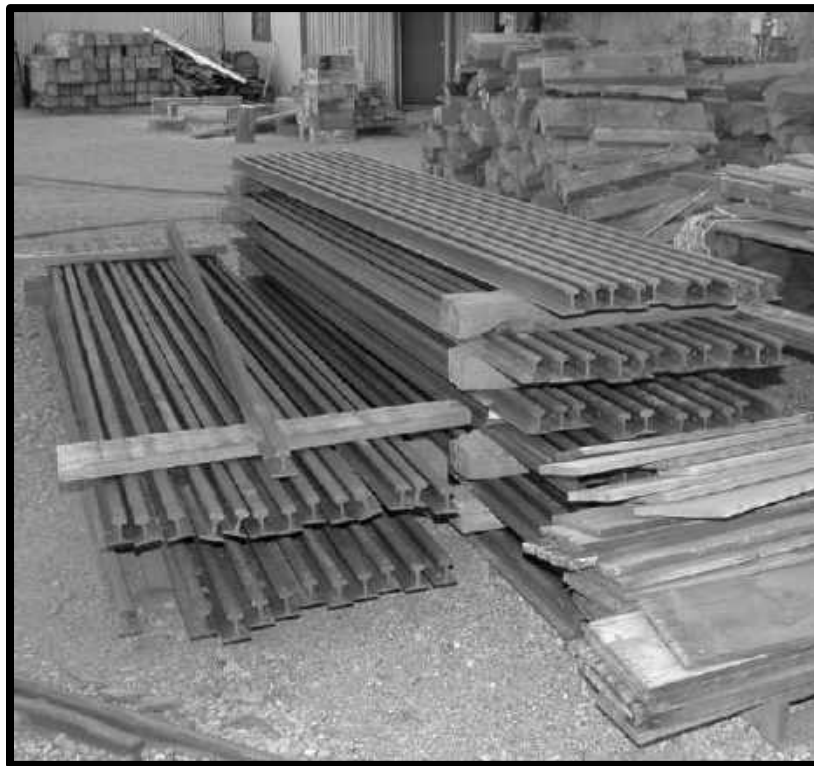
RAIL WAITING TO BE INSTALLED IN THE QUEEN TUNNEL.
