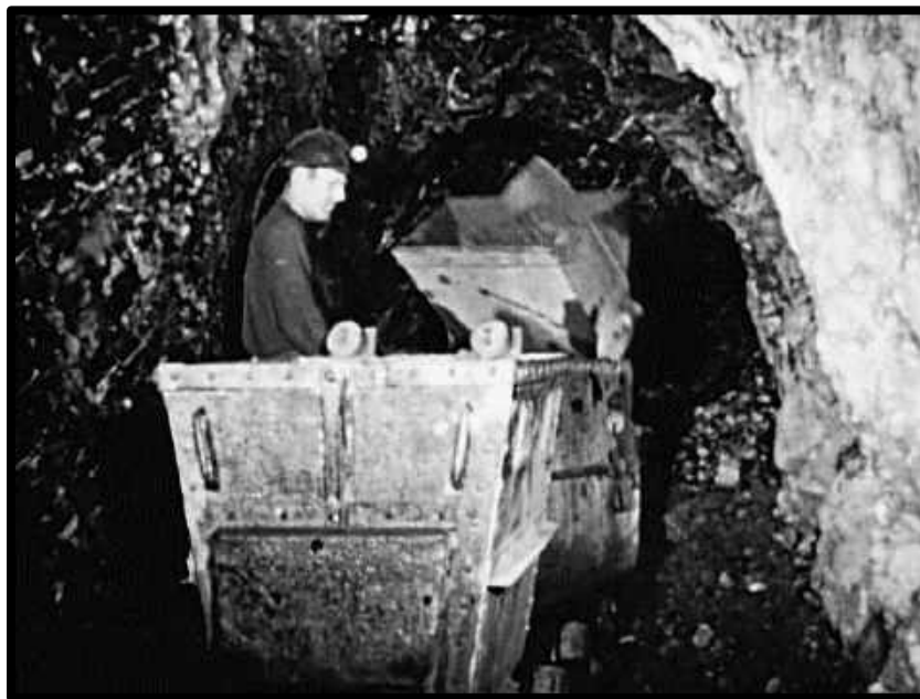
MUCKING WITH A MUCKING MACHINE IN THE CAMPBELL/JUNCTION MINE. C-1940
