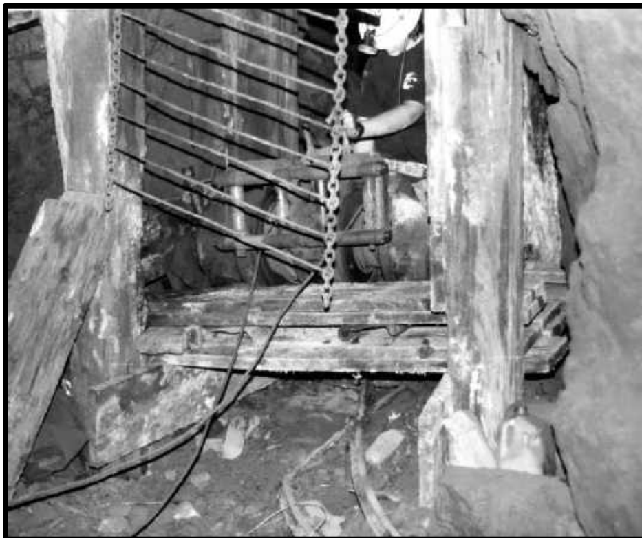
BACKLASH SCREEN WITH SLUSHER ABANDONED ON THE SHATTUCK MINE, 200 LEVEL.
