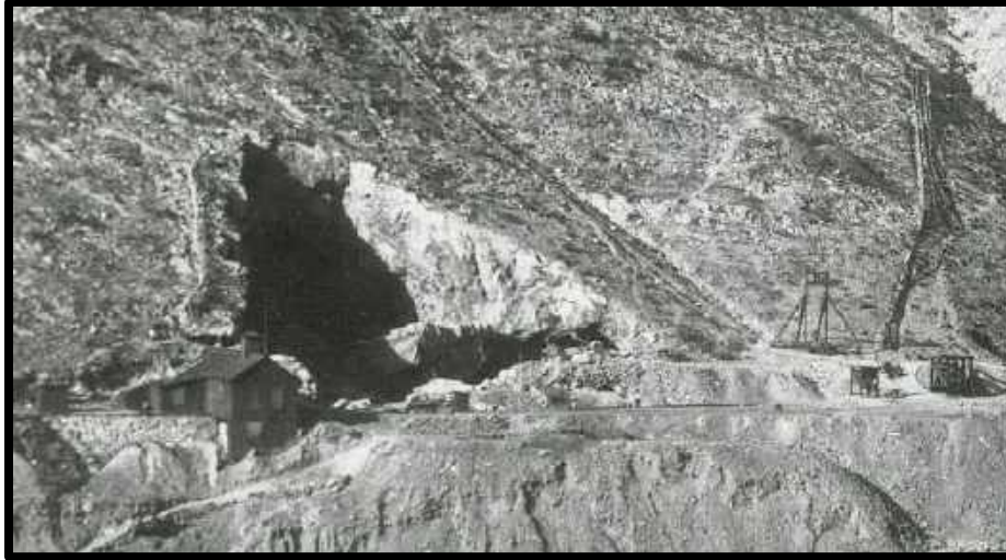
COPPER QUEEN MINE BUILDING ARE THE HOISTING WORKS OF THE INCLINE SHAFT ON THE LEFT WITH THE OPEN CUT (GLORYHOLE) TO THE RIGHT. THE SMALL HEADFRAME IS THE WEST SHAFT C-1900
