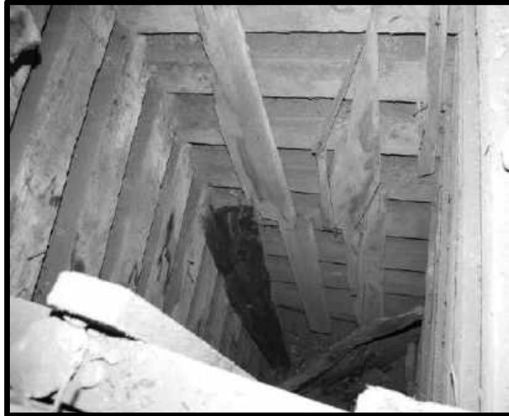
CRIBBED RAISE (ABANDONED) IN THE COPPER PRINCE MINE.
