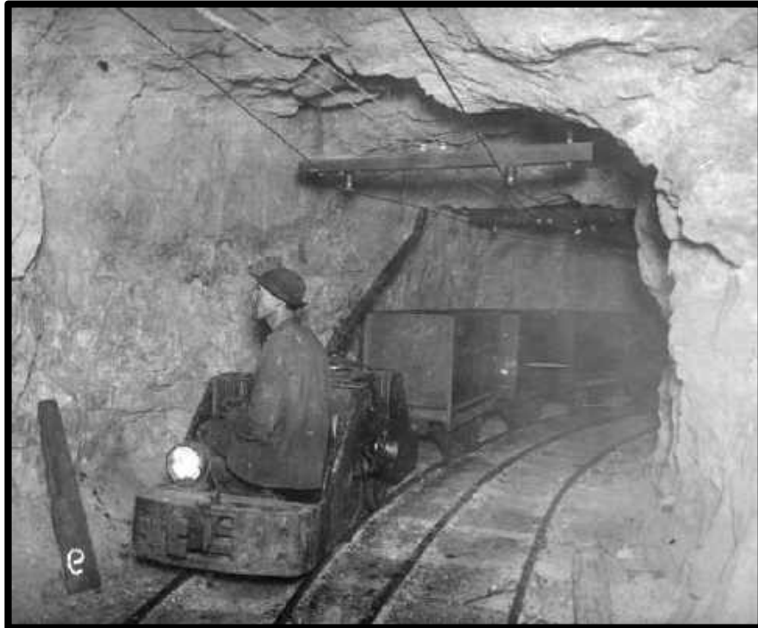
TROLLEY PULLING GABLE BOTTOM MINE CARS. C-1910
