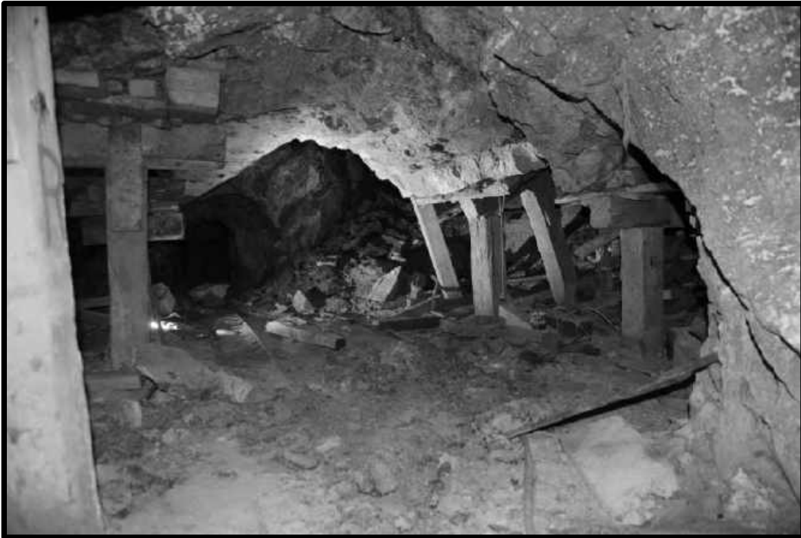
STOPE (DEF.1) HIGGINS MINE, TUNNEL LEVEL.
