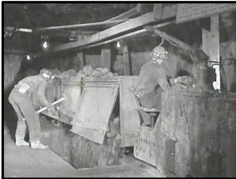
GABLE-BOTTOM CAR (S) PORPHYRY STYLE BEING DUMPED IN THE JUNCTION MINE C-1938
