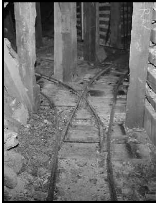
KICK SWITCH ON THE 1 ST LEVEL OF THE HARGIS INCLINE
