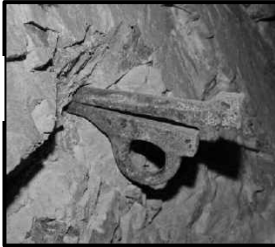
EYE BOLT WEDGE STYLE, 3 RD LEVEL, SOUTHWEST MINE
