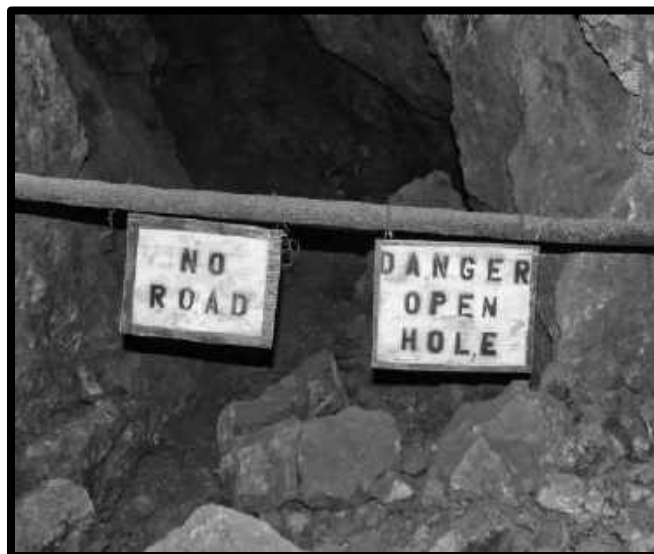
OPEN HOLE POSTED IN THE COPPER PRINCE MINE
