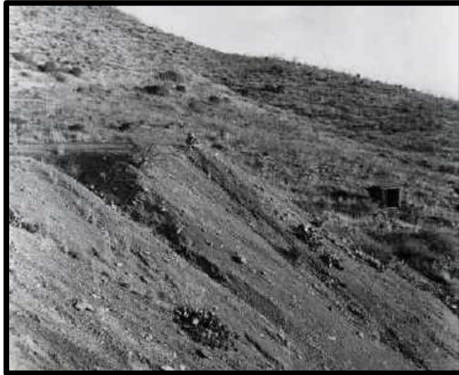
ANGLE OF REPOSE IS SHOWN BY THE DUMP OF THE ABANDONED, LAKE SUPERIOR & PITTSBURG #3 SHAFT c-1960's
