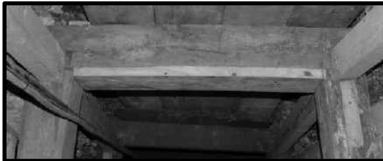
SPREADER SCAB 30 CROSSCUT, 3 RD LEVEL, SOUTHWEST MINE.
