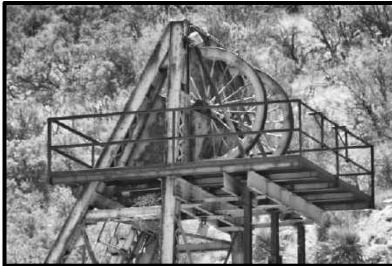
SHEAVE WHEEL(S) A TOP THE SHATTUCK MINE HEADFRAME.
