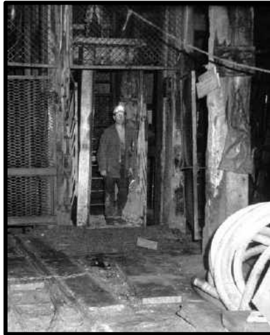
BULL HOSE (LOWER RIGHT) ON THE 1450 LEVEL STATION OF THE COLE SHAFT
