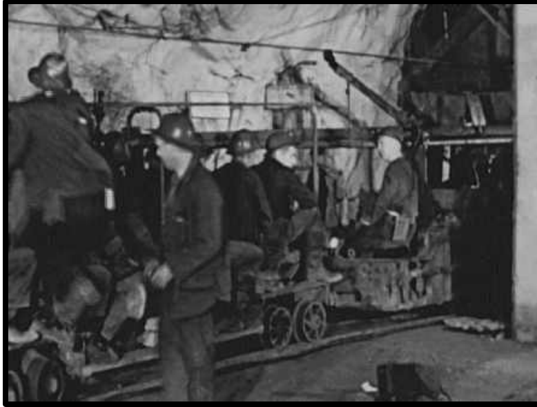
MAN CAR ON THE 2966 STATION OF THE CAMPBELL MINE.
