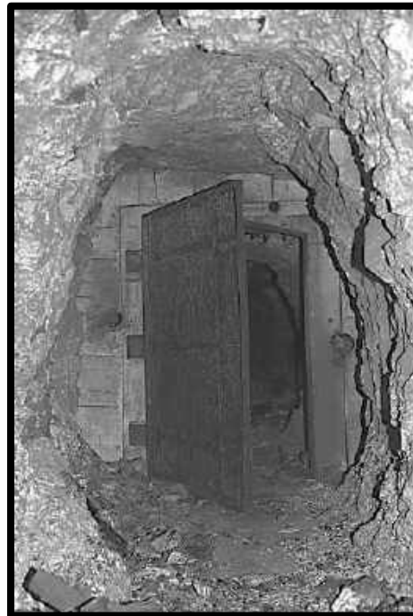
FIRE DOOR ON THE 6 TH LEVEL STATION OF THE SUNRISE SHAFT.
