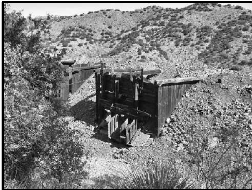
ORE BIN(S) AT THE HIGGINS MINE.
