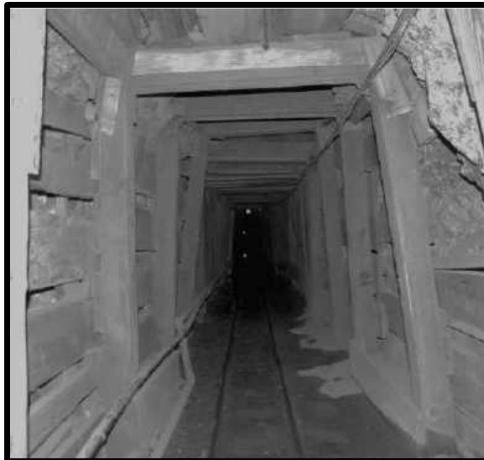
DRIFT SET(S) 30 CROSSCUT, 3 RD LEVEL, SOUTHWEST MINE
