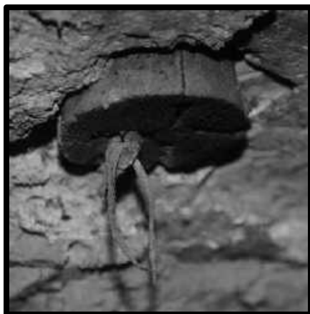
SPAD IN THE CEILING (BACK) OF A CROSSCUT ON THE 6TH LEVEL SOUTHWEST MINE.
