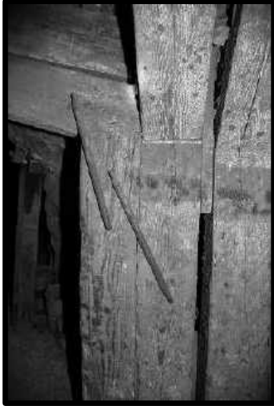
TIMBER DOGS , LEFT AT 3 RD LEVEL STATION OF THE SOUTHWEST MINE. RIGHT, STORED ON A PALLET AT THE QUEEN MINE TOUR.
