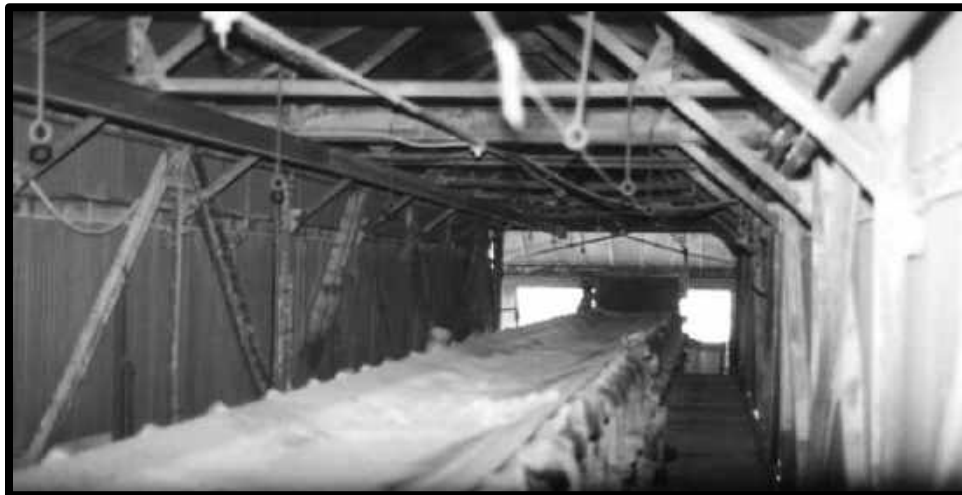
BELT ON THE DALLAS MINE CONVEYOR
