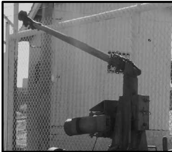
TROLLEY POLE ON A PUP MOTOR AT THE JUNCTION MINE GATE
