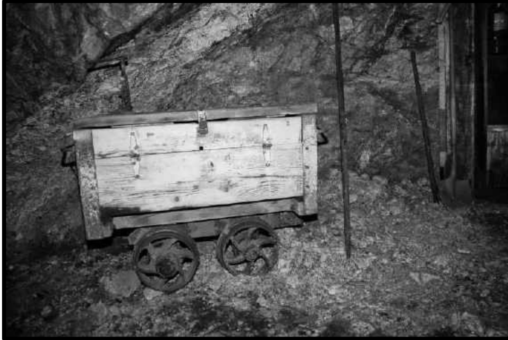
PIPE AND TRACK CAR 86 CROSSCUT, 3 RD LEVEL, SOUTHWEST MINE.
