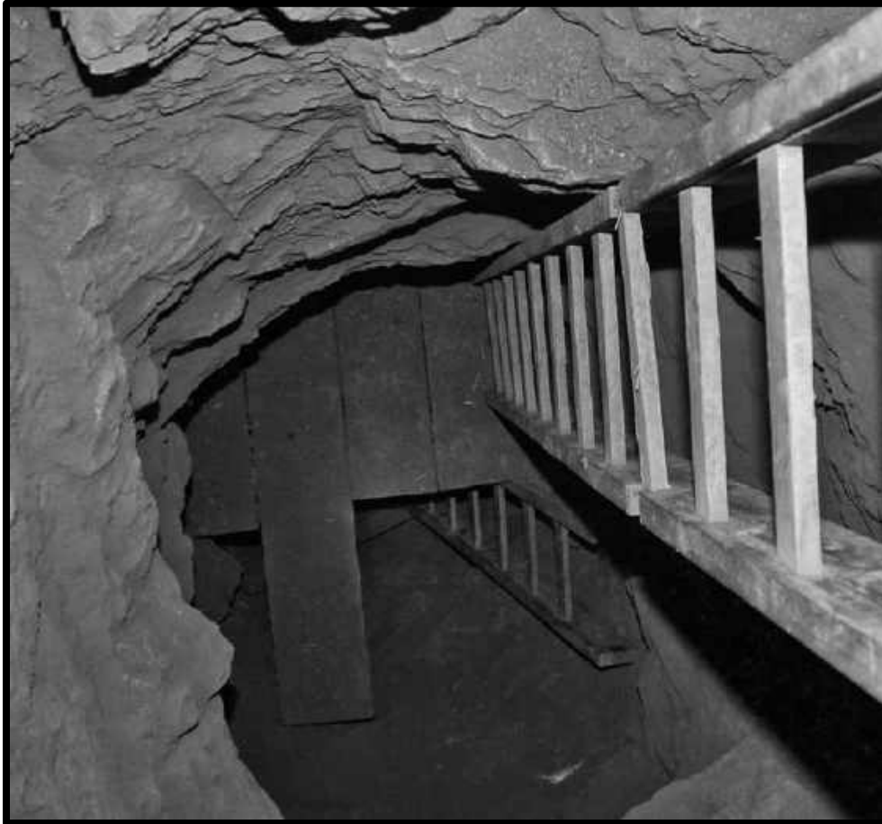
LANDING IN A MANWAY BETWEEN 64 CROSSCUT ON THE 3 RD LEVEL SOUTHWEST MINE AND THE COPPER PRINCE MINE
