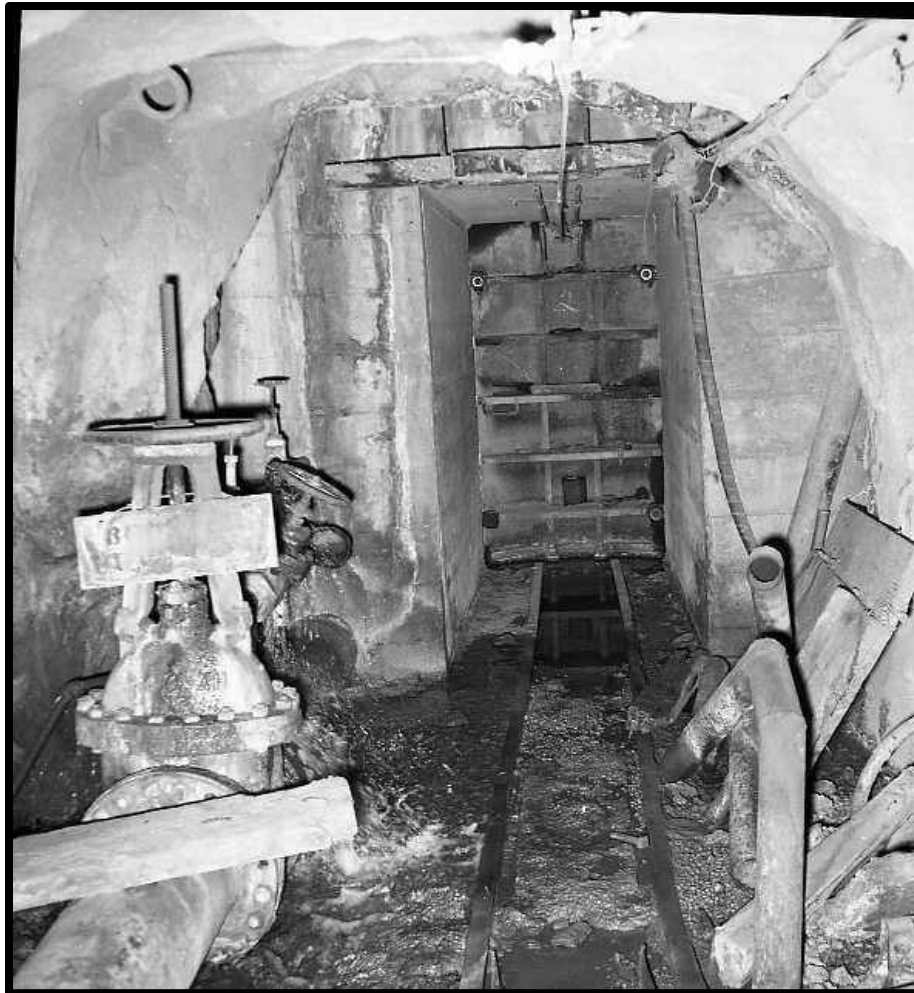
WATER DOOR CAMPBELL MINE, 12 CROSSCUT, 2700 LEVEL.
