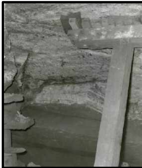
SLABBY GROUND IN A STOPE THE MINE IS UNKNOWN C-1955
