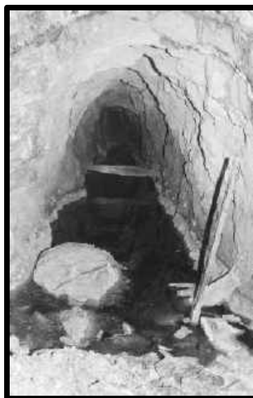
ACID MINE WATER SOUTHWEST MINE, 6 TH LEVEL, 16 CROSSCUT, WEST OF 32 CROSSCUT
