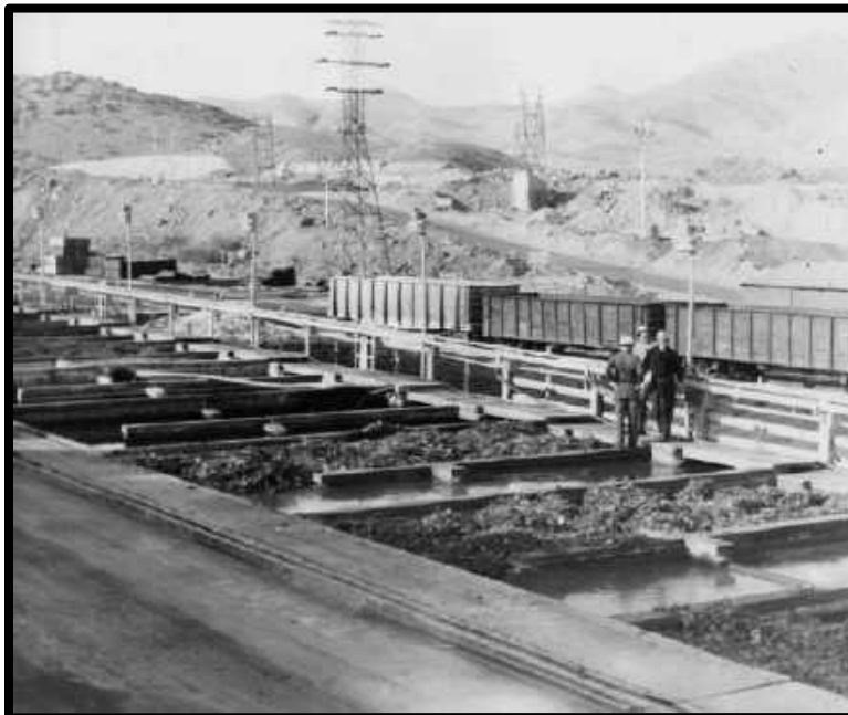
PRECIPITATION PLANT AT THE CAMPBELL MINE C-1955
