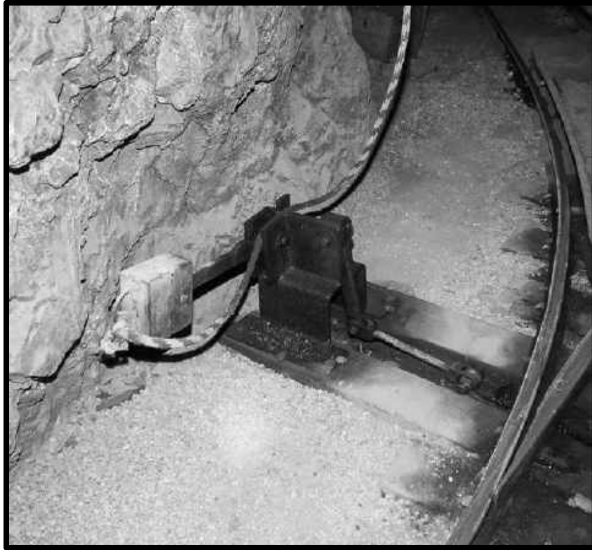
SWITCH THROW AT THE INTERSECTION OF 30 AND 35 CROSSCUTS ON THE 3 RD LEVEL SOUTHWEST MINE.
