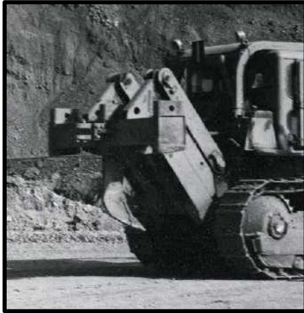
RIPPER ON A CATERPILLAR BULLDOZER IN THE LAVENDER PIT C-1960
