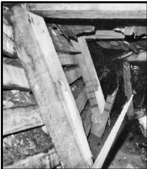
KICKED OUT POSTS ON THE 7 TH LEVEL SOUTHWEST MINE
