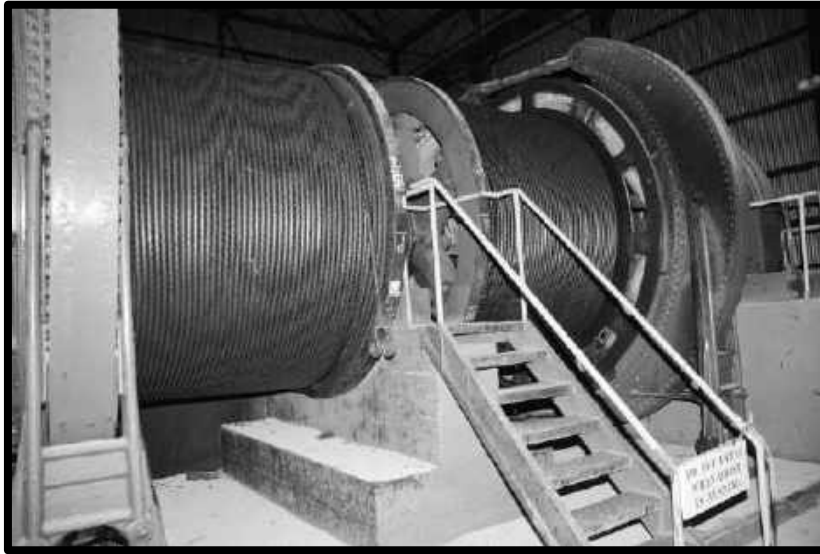
CABLE ON THE DALLAS MINE ORE HOIST.
