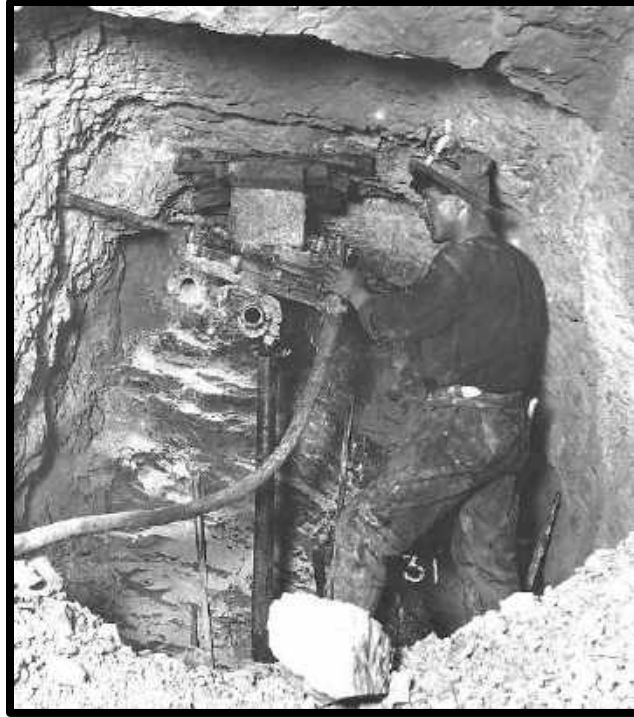
WIDOW MAKER AN INGERSOLL-SERGEANT, DRY DRILL NOTE IT ONLY HAS A COMPRESSED AIR HOSE AND NO WATER HOSE GOING TO THE DRILL. IN AN UNKNOWN MINE IN BISBEE C-1903
