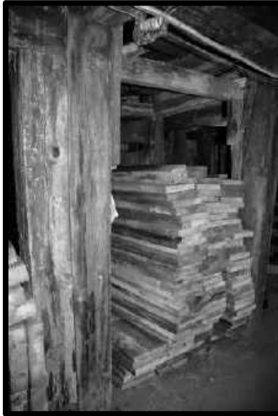
LAGGING STACKED IN A TIMBER STATION AT THE COPPER QUEEN INCLINE 3 RD LEVEL SW. STATION.
