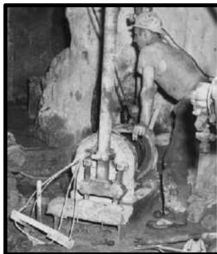
AIR HOIST BEING OPERATED AT A CALYX DRILL. C1960'S
