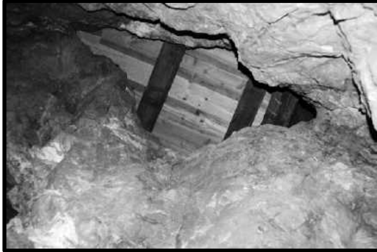
BULKHEAD IN THE BACK (CEILING) OF A STOPE WHERE IT WAS INTERSECTED BY AN INCLINED RAISE. COPPER PRINCE MINE
