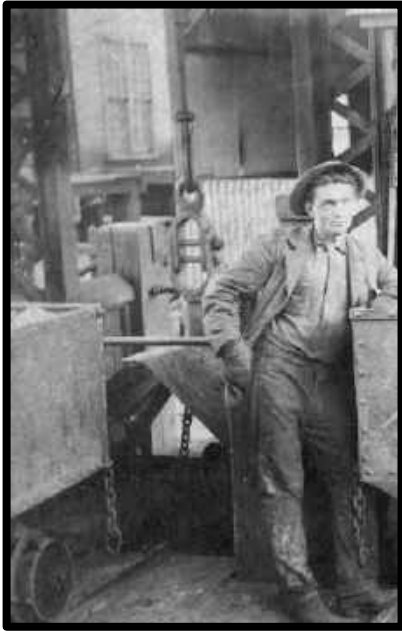
CAGE END OF A CABLE CAN BE SEEN BEHIND THE MINER. IN THIS EXAMPLE CABLE CLAMPS SECURE THE CABLE TO THE CAGE C-1905
