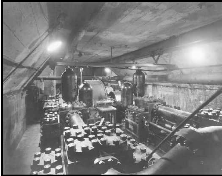
PUMP STATION ON THE 2200 LEVEL OF THE JUNCTION MINE
