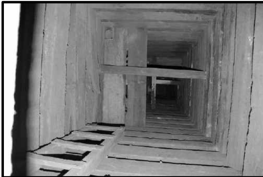
MANWAY LOOKING UP 4-26 RAISE, 4 TH LEVEL, SOUTHWEST MINE. NOTE THE NEXT LADDER IS MISSING.
