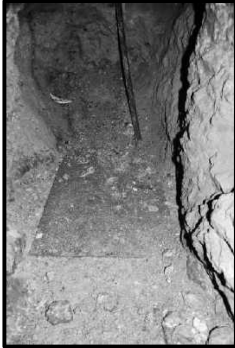
MUCK SHEET IN A DRIFT OFF 55 CROSSCUT ON THE 5 TH LEVEL SOUTHWEST MINE.
