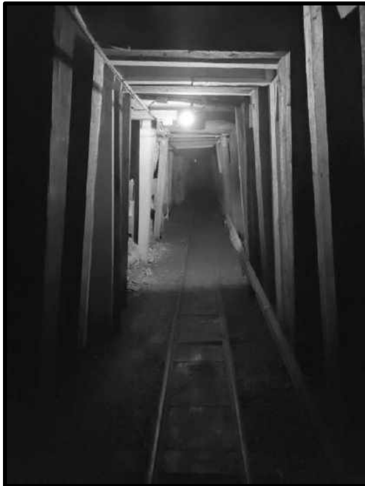
SQUARE TIMBER USED TO BUILD DRIFT SETS 30 CROSSCUT, 3 RD LEVEL, SOUTHWEST MINE.
