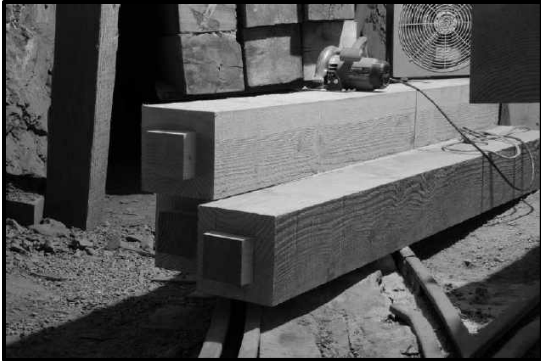
FRAMING TENONS ON POSTS, 3 RD LEVEL SOUTHWEST MINE AT THE INTERSECTION OF 30 AND 35 CROSSCUTS.
