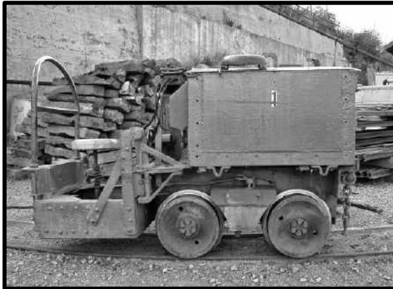
MANCHA MOTOR AT THE QUEEN TUNNEL PORTAL.
