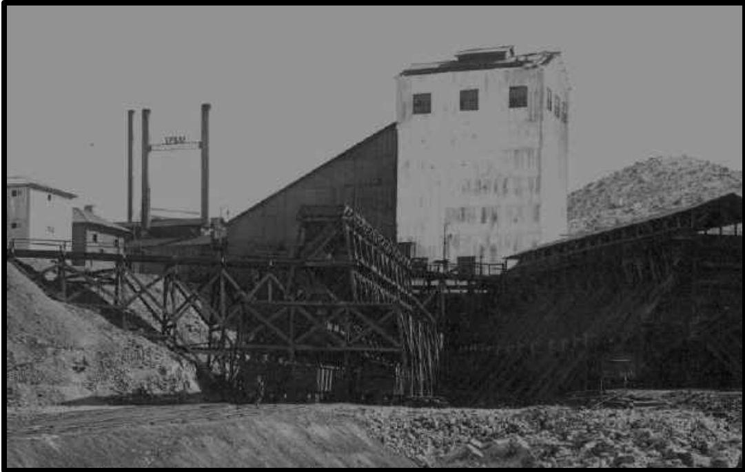
ENCLOSED HEADFRAME AT THE SPRAY MINE
