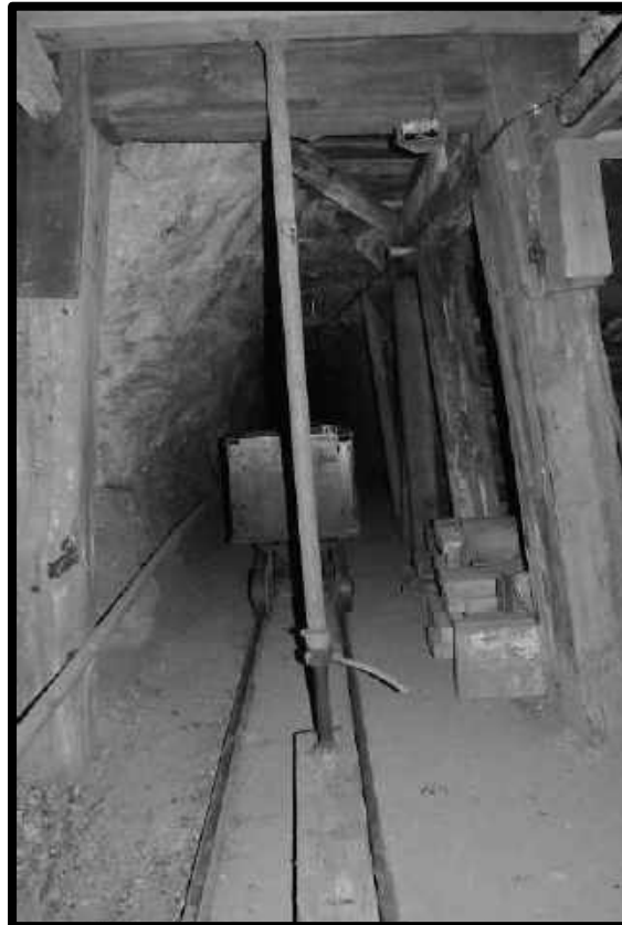
TIMBER JACK AT THE COPPER QUEEN SHAFT 3 RD LEVEL SW. STATION, DURING RETIMBERING
