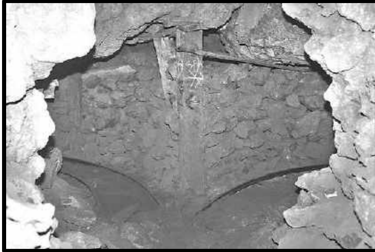
GOB WALL (S) AT AN INTERSECTION OF 2 CROSSCUT ON THE 5 TH LEVEL SOUTHWEST MINE.
