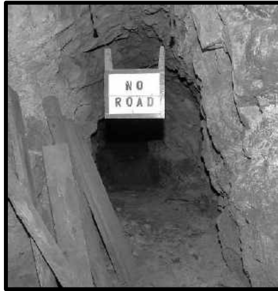
NO ROAD SIGN IN 39 CROSSCUT 3 RD LEVEL SOUTHWEST MINE.
