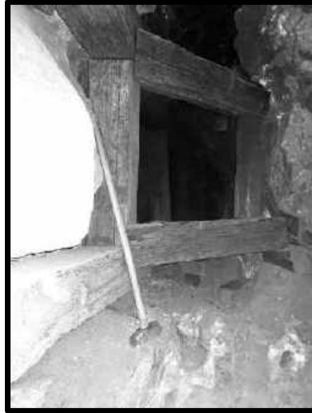
DOG HOLE IN THE RIB OF A STOPE. B LEVEL COPPER QUEEN MINE
