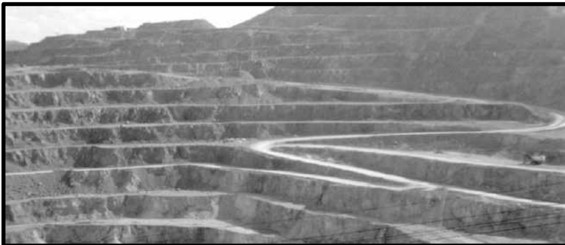
RAMP (DEF.2) LEADING OUT OF THE LAVENDER PIT.
