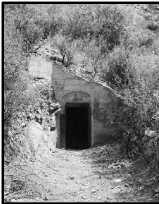
SOUTHWEST TUNNEL PORTAL IN HENDRICKS GULCH.
