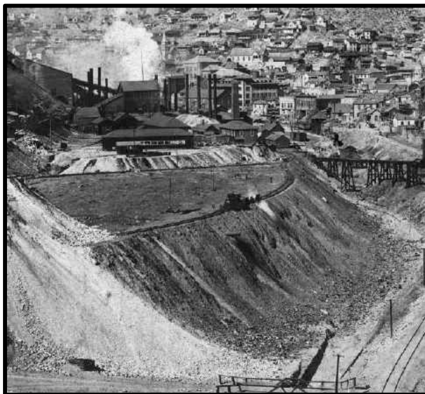
SLAG BEING DUMPED. THE SMELTER AND CZAR MINE ARE IN THE BACKGROUND C-1902
