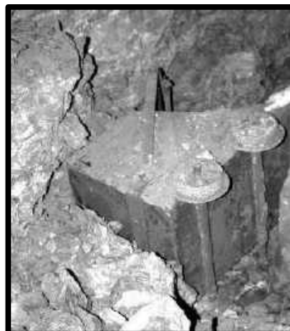
SKIP (ABANDONED) AT THE TOP OF THE WOLVERINE INTERIOR SHAFT IN THE WOLVERINE COUNTRY OF THE HIGGINS MINE
