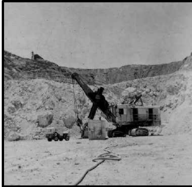
SHOVEL (DEF.2) ELECTRIC SHOVEL IN THE LAVENDER PIT BELOW THE GARDNER SHAFT.
