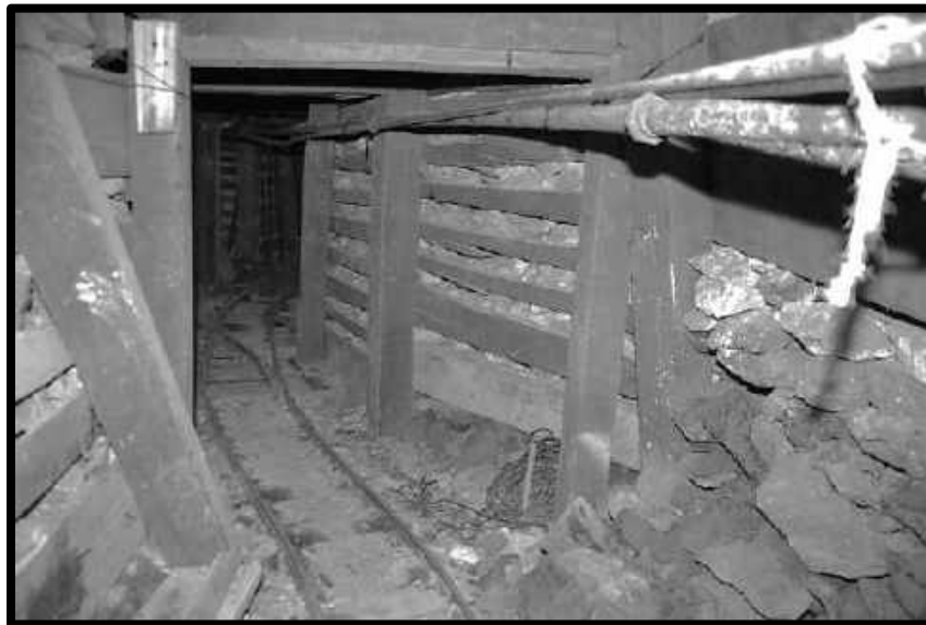
GOB FENCE ON THE 1 ST LEVEL OF THE HARGIS INCLINE
