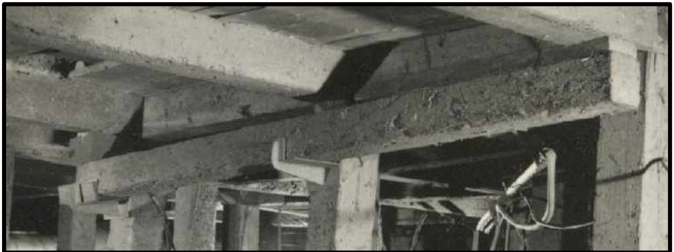
SIDE BOOM HANGER(S) IN THE CAMPBELL MINE.
