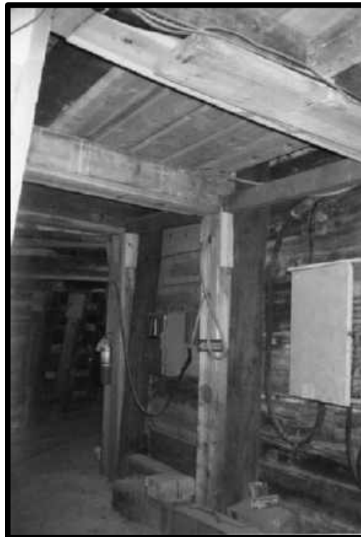
BACK LAGGING, JUNCTION MINE, 770 LEVEL, STATION
