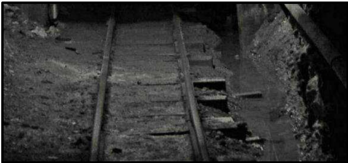
WATER DITCH ON RIGHT SIDE OF RAILS.
