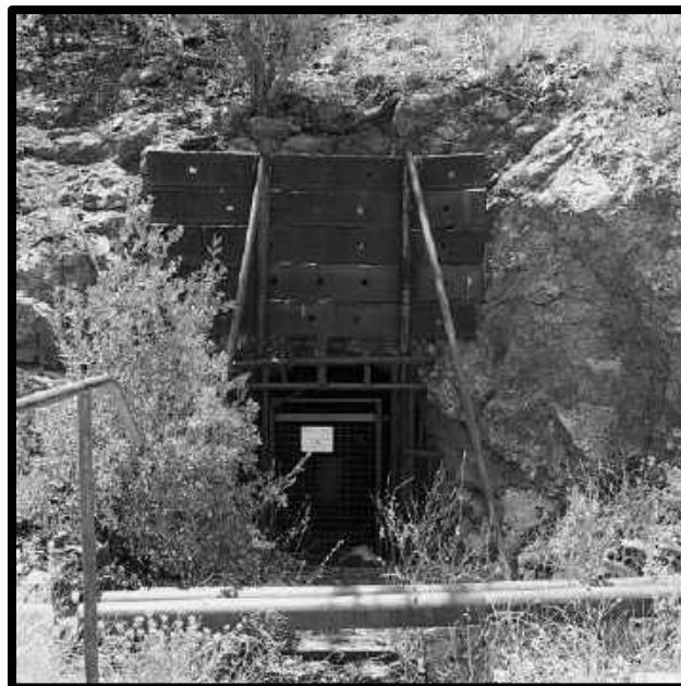
PORTAL OF THE SHATTUCK ADIT
