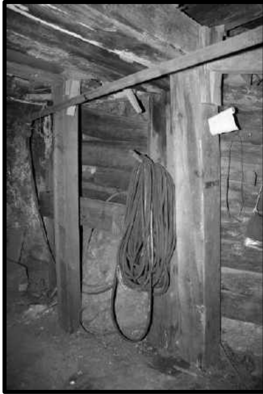
WATER HOSE IN 61 CROSSCUT, 3 RD LEVEL, SOUTHWEST MINE.
