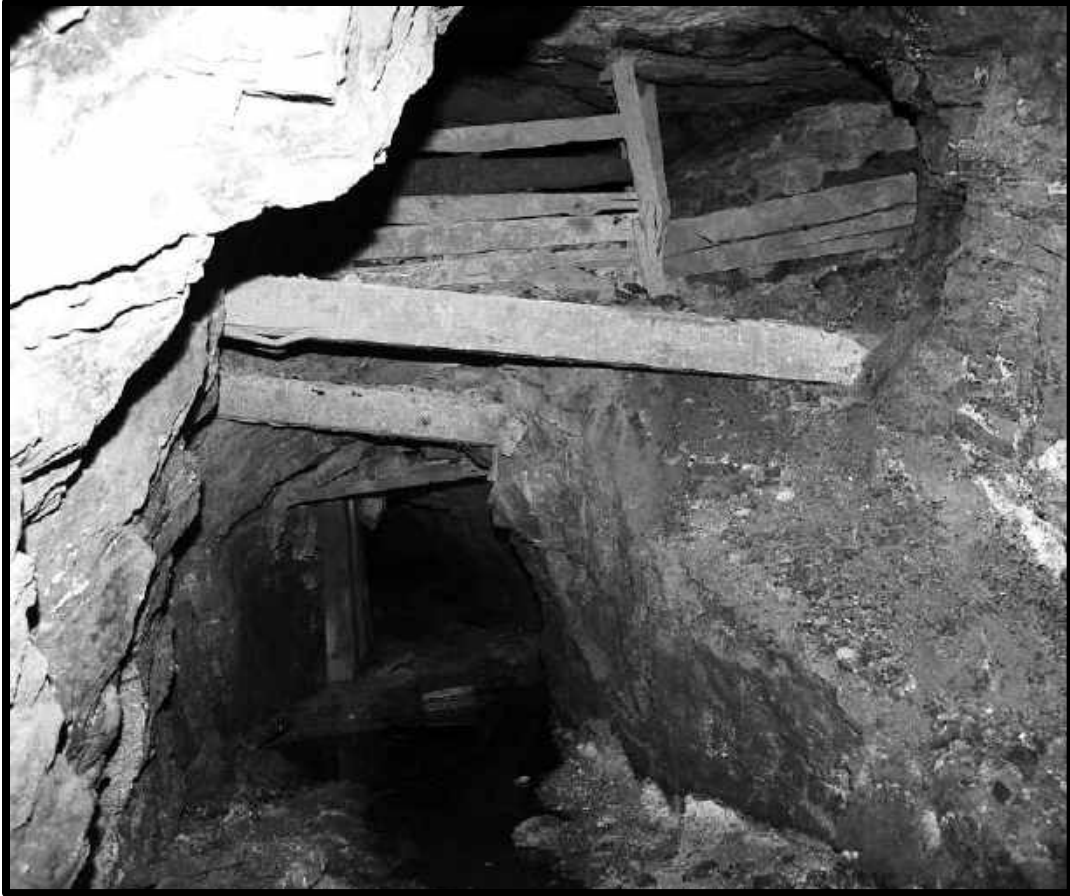
STRINGER 6 TH LEVEL SOUTHWEST MINE
