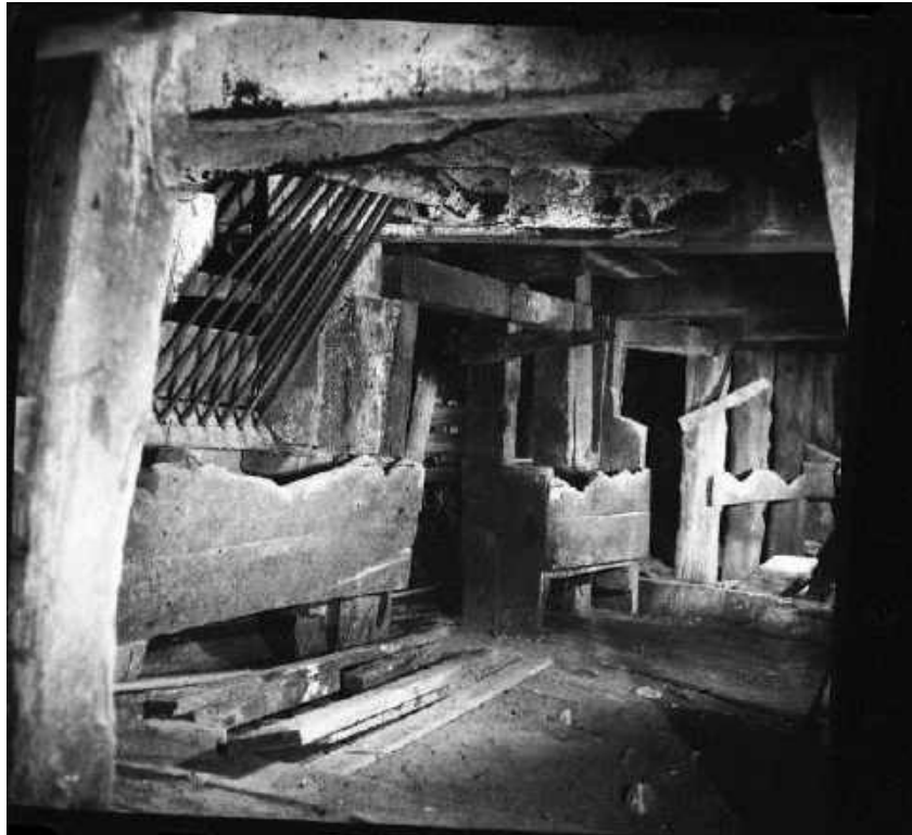
MULE BARN (ABANDONED) ON THE 1500 LEVEL OF THE JUNCTION MINE.
