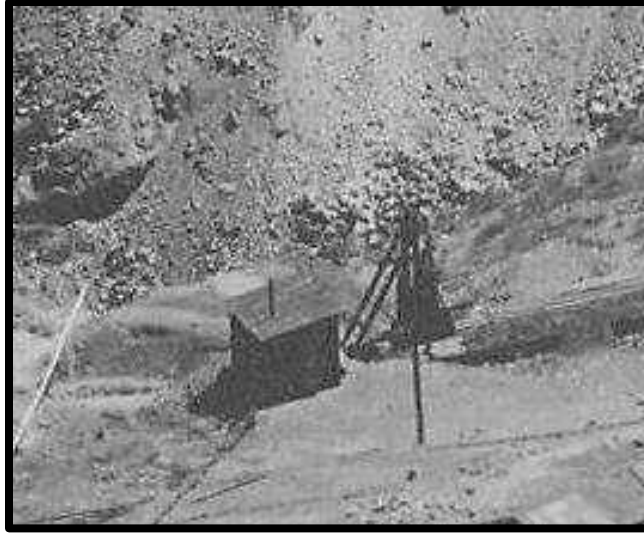
VENTILATION SHAFT IN THE HOLBROOK MINE AREA. C-1925
