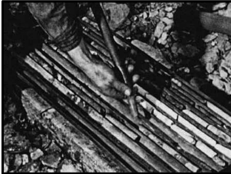
CORE BEING REMOVED FROM A CORE BARREL AND BEING PLACED INTO A CORE TRAY. JUNCTION OR CAMPBELL MINE C-1940
