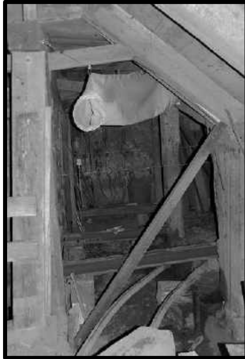
VENT BAG AT THE 3 RD LEVEL SOUTHWEST SHAFT STATION, DURING RETIMBERING.
