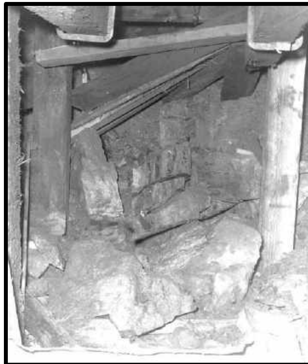
SLABBED THE SITE, H. ORTON WAS SLABBED ON MARCH 14, 1967 IN 31-B STOPE ON THE 3100 LEVEL CAMPBELL MINE. HE SURVIVED WITH, BUT WAS STRUCK WITH SUCH FORCE HIS WHEAT LAMP MARK II WAS TORN OFF AND CAN BE SEEN IN THE CENTER OF THE IMAGE.
