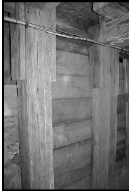
SKIN TO SKIN THE LAGGING ARE PLACED SKIN TO SKIN, 3 RD LEVEL, SOUTHWEST MINE
