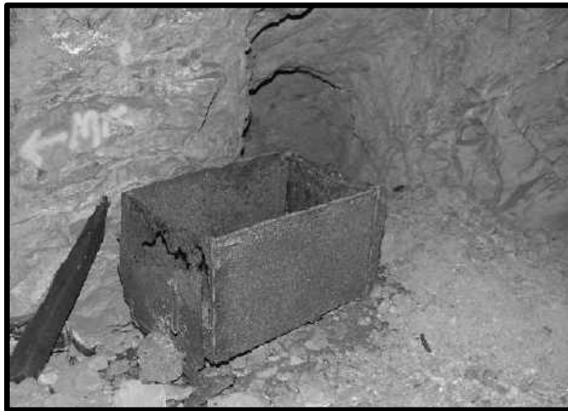
TUB WORN OUT AND RUSTED, 55 CROSSCUT, 5 TH LEVEL, SOUTHWEST MINE.
