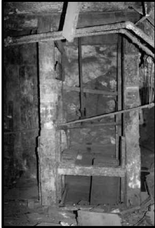
SOUTHWEST SHAFT (#3) ABANDONED; 4 TH LEVEL STATION.
