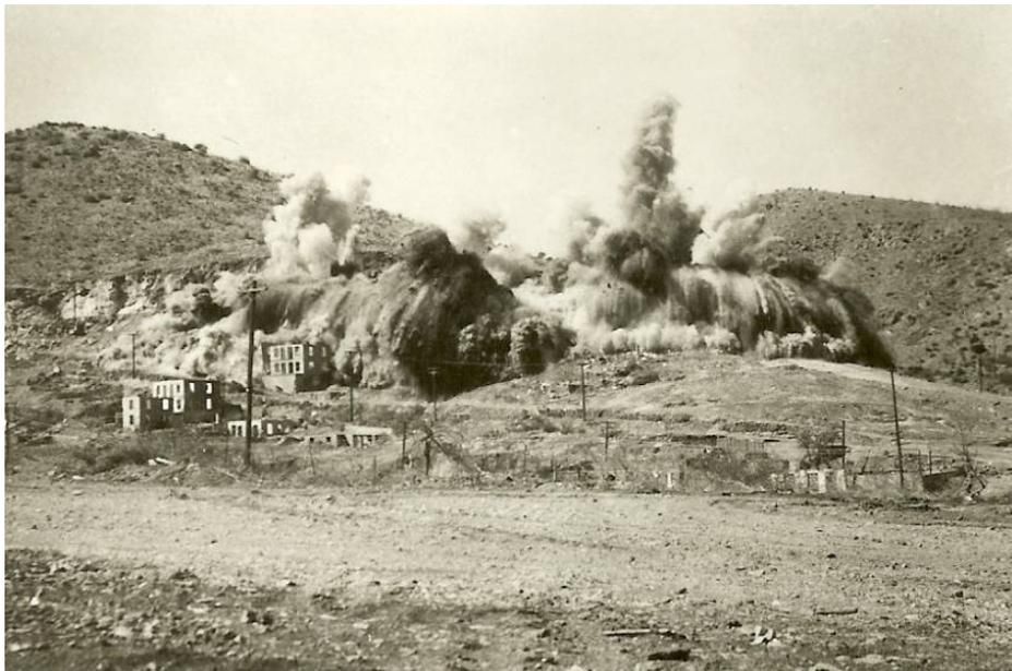
**Figure 4: A photograph of the first blast taking place in what was Johnson Addition, to prepare for the excavation of the Lavender Pit, circa 1950's. To the left of the image, one can clearly see the remnants of vacant concrete buildings. These structures apparently could not be moved like hundreds of others which were in order to make way for the development of the new mining project. Graeme-Larkin collection.**
