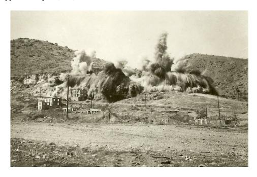
Figure 4: A photograph of the first blast taking place in what was Johnson Addition, to prepare for the excavation of the Lavender Pit, circa 1950's. To the left of the image, one can clearly see the remnants of vacant concrete buildings. These structures apparently could not be moved like hundreds of others which were in order to make way for the development of the new mining project.
