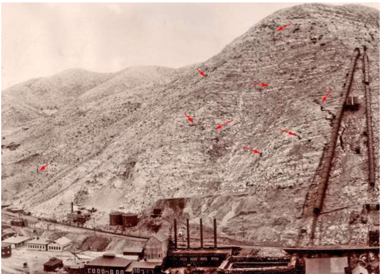
Figure 1.2.29: Queen Hill above the Czar Mine with a few of the numerous subsidence cracks caused by mining activity noted by arrows - 1909. Local lore incorrectly has it that these cracks were the result of a significant earthquake hit the area in 1887.
