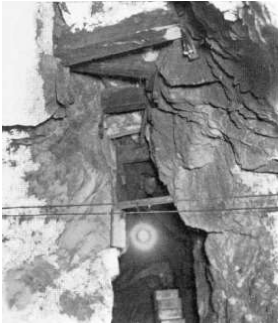
Figure 1.3.2: Fissure on the 200 level, Czar Mine (Douglas, 1900). This was undoubtedly a subsidence caused, marginal crack.
