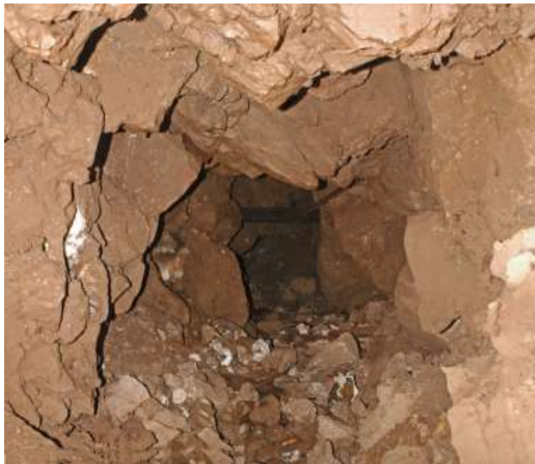
Figure 2.4.6: A crosscut cut through blocky, chaotic boulders of broken limestone showing dilation and breakage along bedding planes, subsequently cemented by minor calcite. This is located more than 100 feet above an oxidation cave and the collapse of the beds was caused by subsidence due to the removal of support below because of oxidation and the formation of a cave. A feature such as this was an important guide to possible ore somewhere below. This is 86 Crosscut on the 6 th level of the Southwest Mine and mining through this broken rock would have been both difficult and dangerous as large blocks of limestone fell from the sides and back (top) . Maximum width - 3.5 meters.
