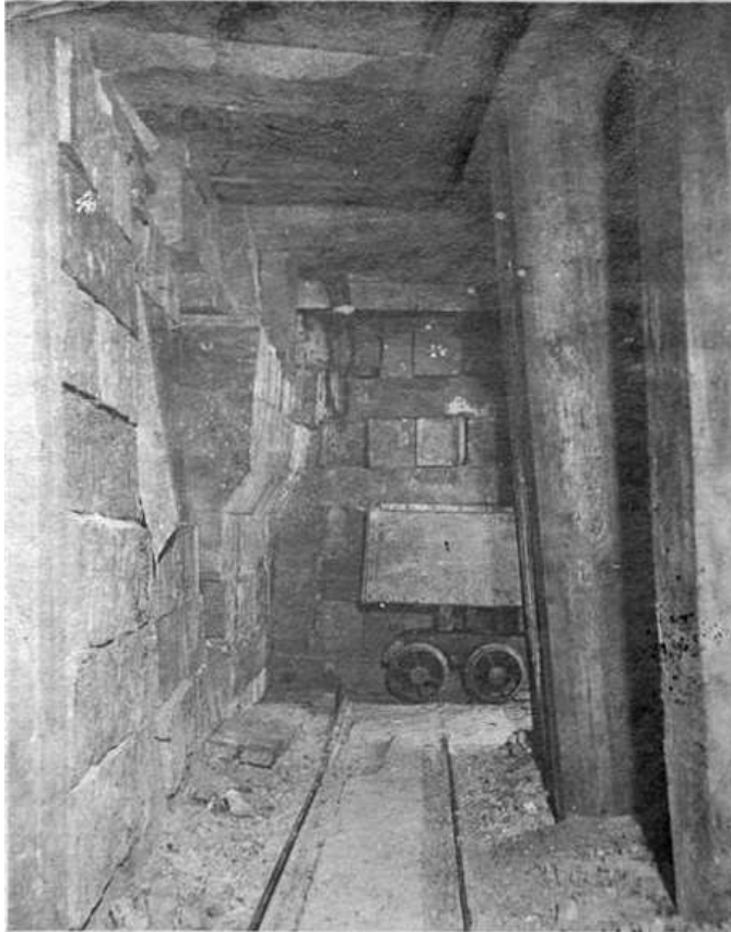
Figure 2.1.3: An example of the timber bulkhead used to keep heavy ground open as described in the 1904 Bisbee Daily Review . The heavy, 25 centimeters by 25 centimeters square timber is actually stacked on top of each other, several layers deep to support the opening. No space could be left open, as the clays would quickly extrude into the workings because of the intense pressure. Holbrook Mine, 1904.
