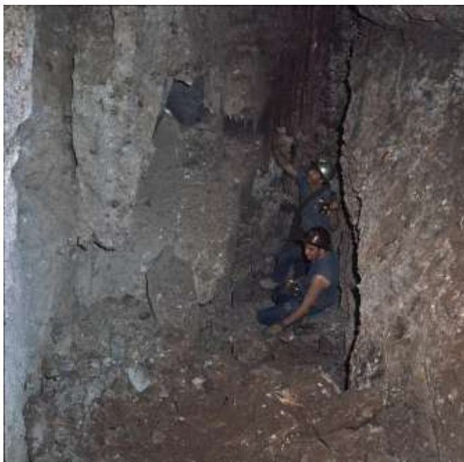
Figure 2.6.2: Cave like opening on the 100 level of the Bisbee Queen Mine in 1967. The right wall is a silica breccia, while the left is limestone. The broken rock in the bottom of the photo is from an exploration working sunk downward for most of 20 meters searching for oxide copper ores that did not exist.
