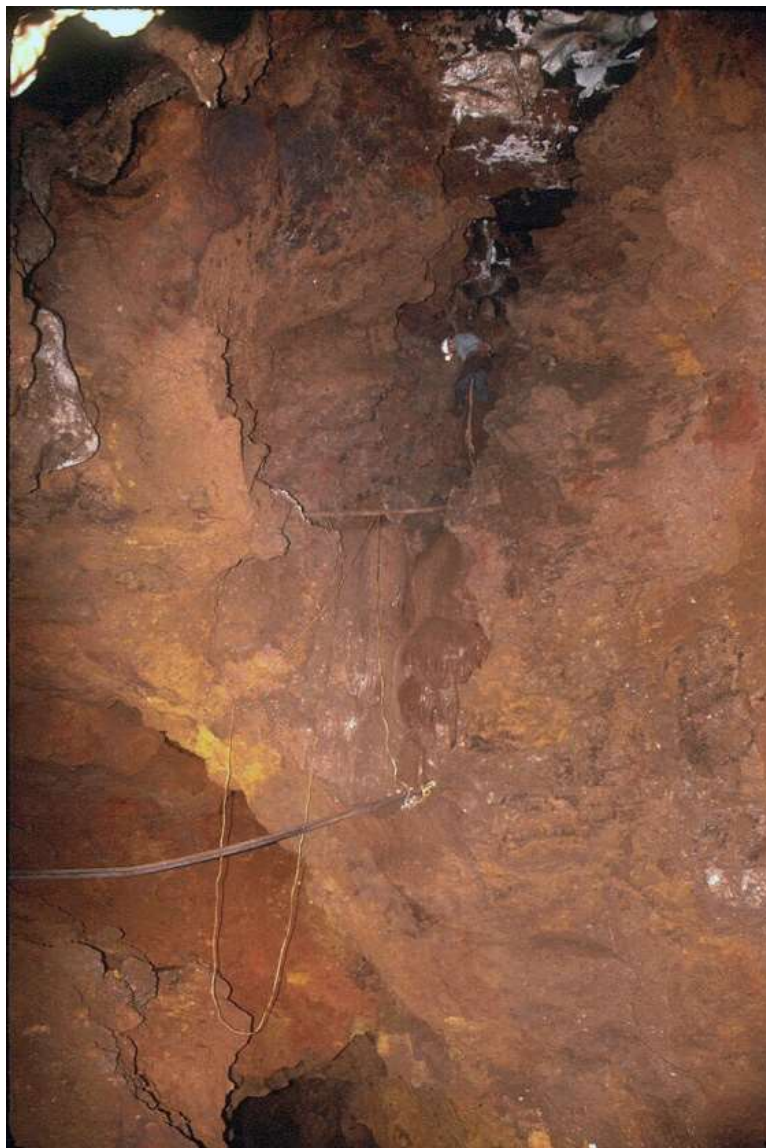
Figure 1.7.11: Descending from the upper part of the cave to the 4 th level. Note the top of the 4 th level drift at bottom center. The calcite at the top is largely white, while that in the center is colored a deep brown. Some limestone is visible as rounded knobs in the left center foreground.
