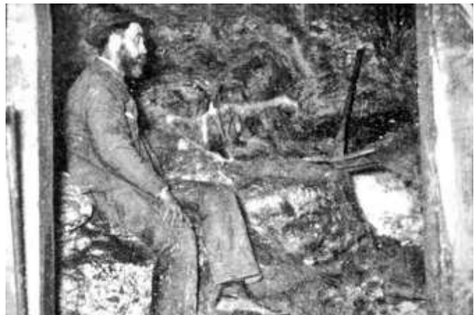
Figure 2.1.1: A face of soft oxide (top) on hard limestone (bottom) in the Czar Mine about 1895. The oxide was so soft it could be removed by just using a pick; no explosives were needed, except to blast the hard limestone. A consequence of this abundant clay, was the need for substantial, heavy timber to support the opening, Douglas (1900).
