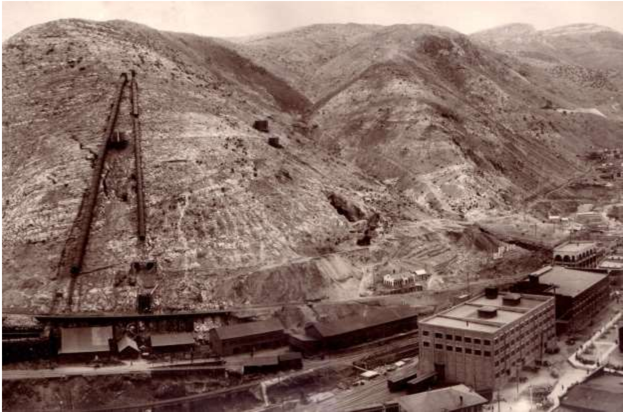
Figure 1.4.1: Queen Hill in 1909. The Southwest Mine exploited Queen Hill, mining rich ores from above the Open Cut of the Copper Queen Mine (center) to the Higgins Mine, seen here in the upper right. The dark area in the upper center of the photo is a silica breccia outcrop adjacent to the huge, New Southwest Orebody, which hosted several important caves.
