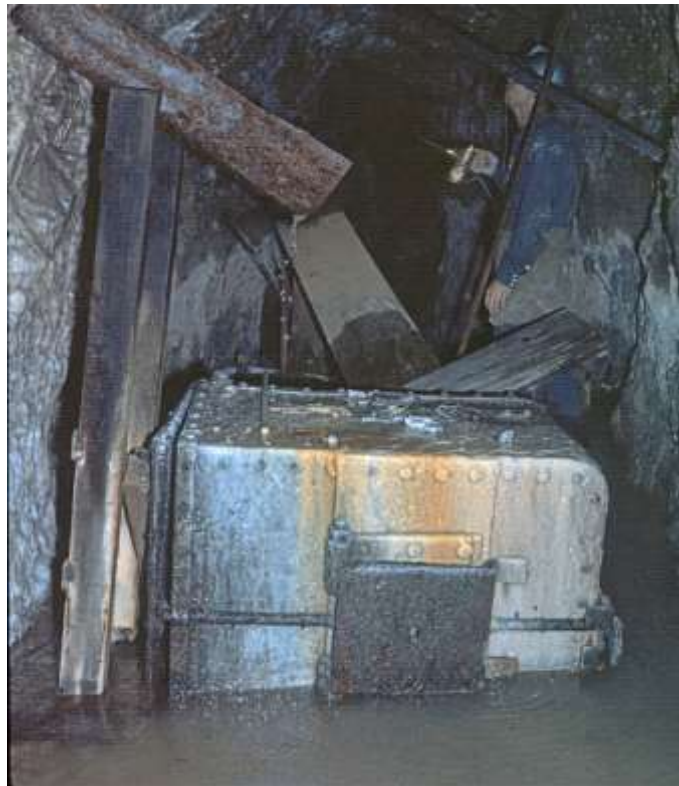
Figure 1.6.1: Post-mining calcite growth on a mine car, Higgins Mine, Tunnel level, 1967. More than 1/2 inch of calcite had been deposited in the just over 20 years since this mine closed. Note the calcite deposition on the left crosscut wall as well. The calcium carbonate rich water is flowing from a small diameter diamond drill prospecting hole.
